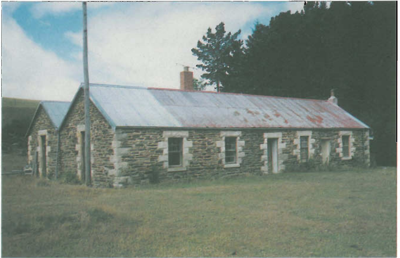
The shearers' quarters at Shag Valley station were more solidly built than the woolshed, using the local schist with quoins and lintels of Oamaru limestone.
