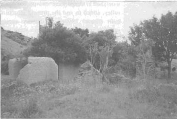
The first house at Rocklands Station had a mud-brick chimney supported by wooden framing. Although the method of construction looks fragile, the chimney has survived for over 120 years.
