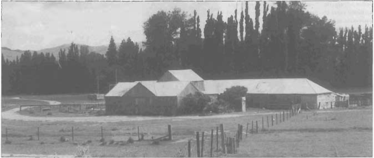
The Blackstone Hill woolshed ( above ) has large corrugated iron extensions around an earlier stone building. The tower for the old screw press still juts above the roofline.
