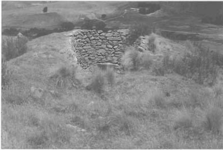
This stone-lined pit, on a hillside above Deep Stream, is the top end of a pressure pipe which once ran down to the hydraulic elevators below, near Rockland Station homestead.
