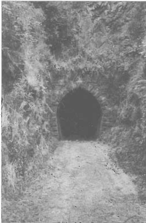
The portal of the Manuka Gorge tunnel on an old branch line to Lawrence.
