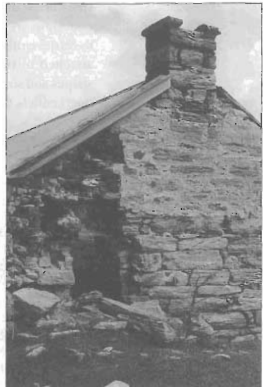
The shearers had their own cookhouse ( below ) out on the paddock behind the woolshed. Their mud-brick bunkhouse used to stand immediately behind the cookhouse. The cookhouse had its own bread oven ( right ). The collapse of the outer wall shows that the oven was made like a small brick kiln.
