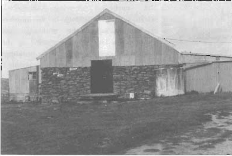
In the 1860s Teviot Station built a U-shaped stone wall. It sheltered shearers when they were working on the far side of the Clutha River from the main shearing shed. When the station was subdivided, corrugated iron was added to make this woolshed, still standing above the Roxburgh Gorge.
