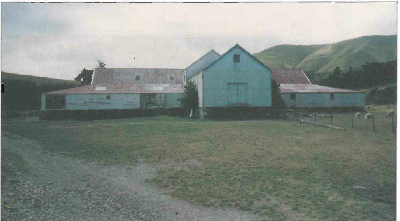
The Shag Valley station woolshed, built in the 1860s, is one of the oldest wooden and corrugated-iron woolsheds in Otago. It could accommodate 40-50 shearers, but the woolroom was relatively small.
