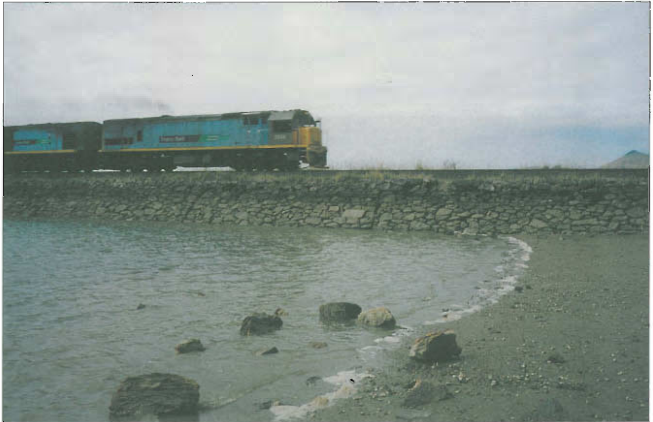
Although this causeway crossing Blanket Bay was built about 1937, when the railway line was shifted and straightened, it is supported by the same sort of hand-stacked walling used around the Otago Harbour since the 1860s.
