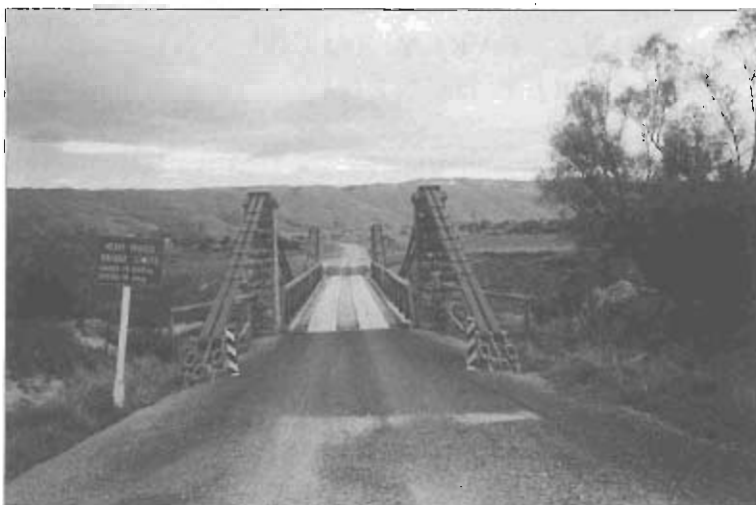
The early road bridges to the gold fields were often suspension bridges with piers built from the local stone. This one is across the Taieri River near Sutton.
