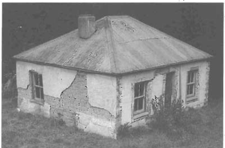
This mud brick house at Macraes was built by Gay Tan, a Chinese miner married to a European woman. The plaster over the mud bricks has been decorated around the front door. Photograph: Peter Bristow
