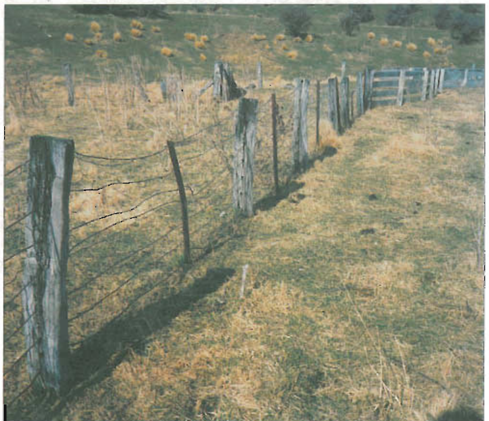
This was one of the first wire fences in Otago, built in the early 1870s at Longlands on the Maniototo, using kowhai posts brought up from Goodwood.
