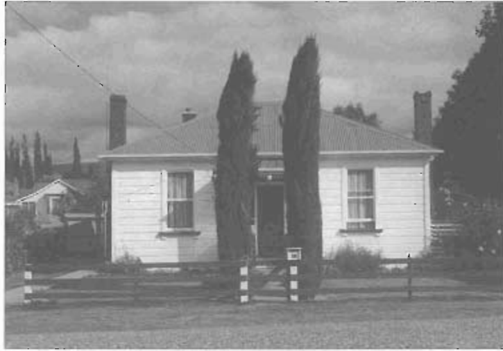
Georgian symmetry remained popular right through to the turn of the century, which is probably when this cottage was built in Lawrence.
