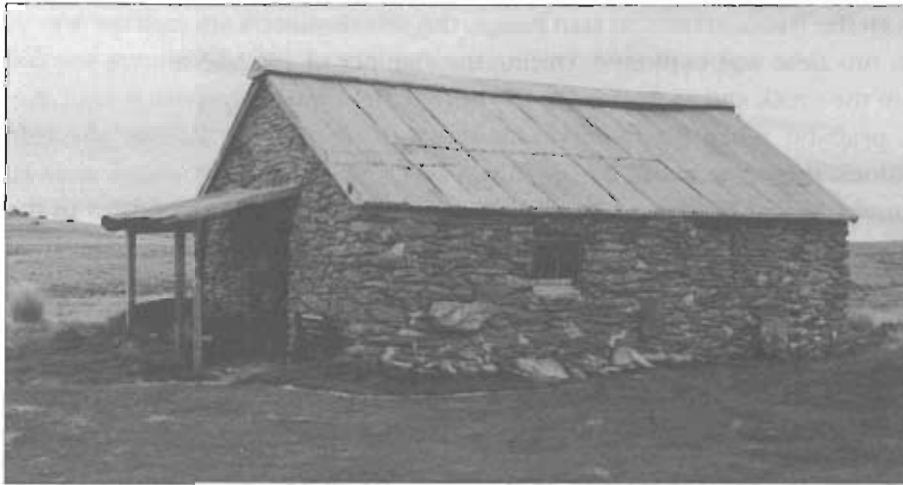
The Serpentine Church was built in 1873 at 1000 m a.s.l. Now owned by the Department of Conservation, its stone walls have been stabilised to last another 120 years. Photograph: Peter Bristow
