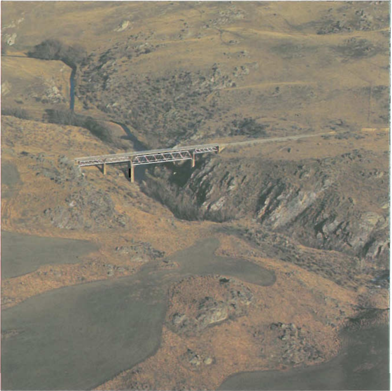
The Poolburn viaduct on the Central Otago Rail Trail. It is an American-type iron trestle bridge on piers of local schist stone, quarried from nearby. Photograph: Kevin Jones, DOC
