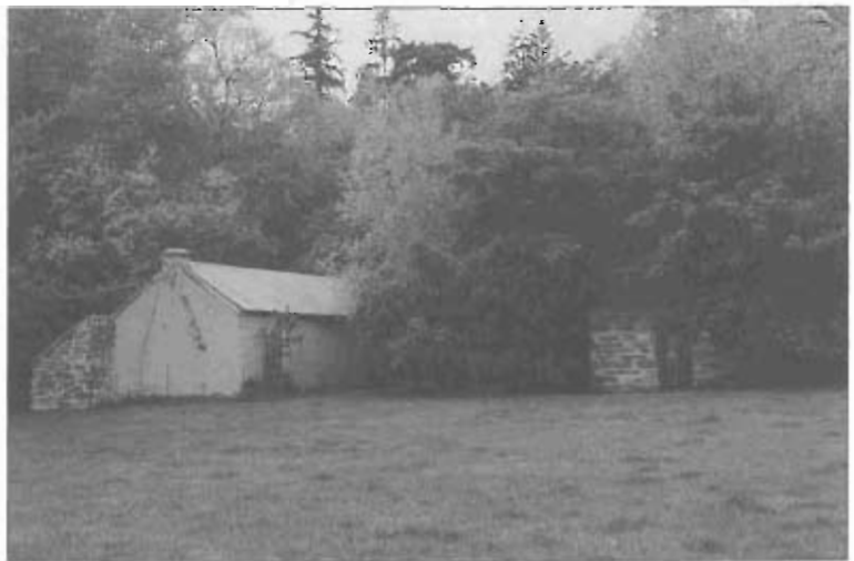
The Blackstone Hill woolshed ( above ) has large corrugated iron extensions around an earlier stone building. The tower for the old screw press still juts above the roofline.
