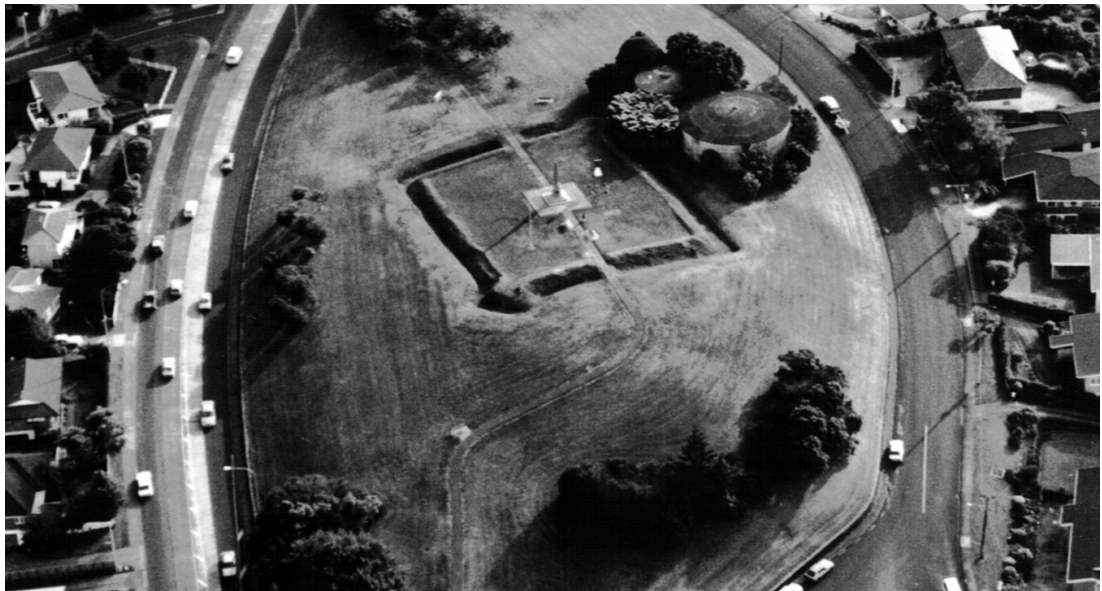
Figure 21. Howick Stockade; the defensive ditch outside the stockade defence has been subject to reconstruction. Photo: N. Prickett, 1992.
