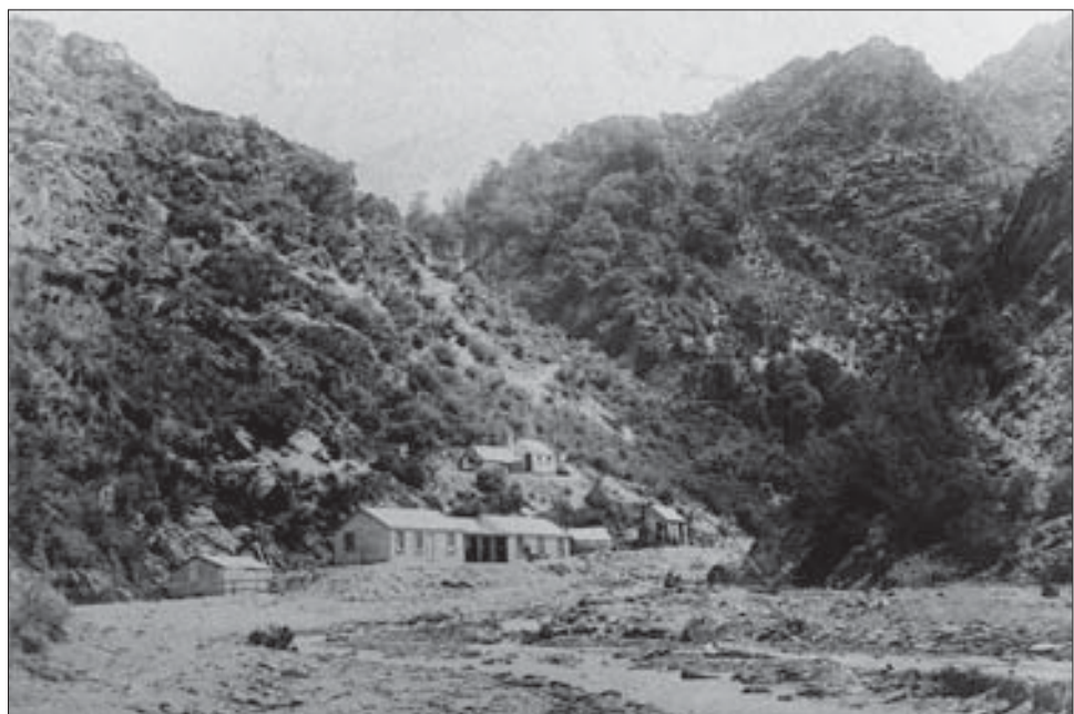
Figure 37. Phoenix Hotel, looking up Skippers Creek. Photo: Hocken Library.
