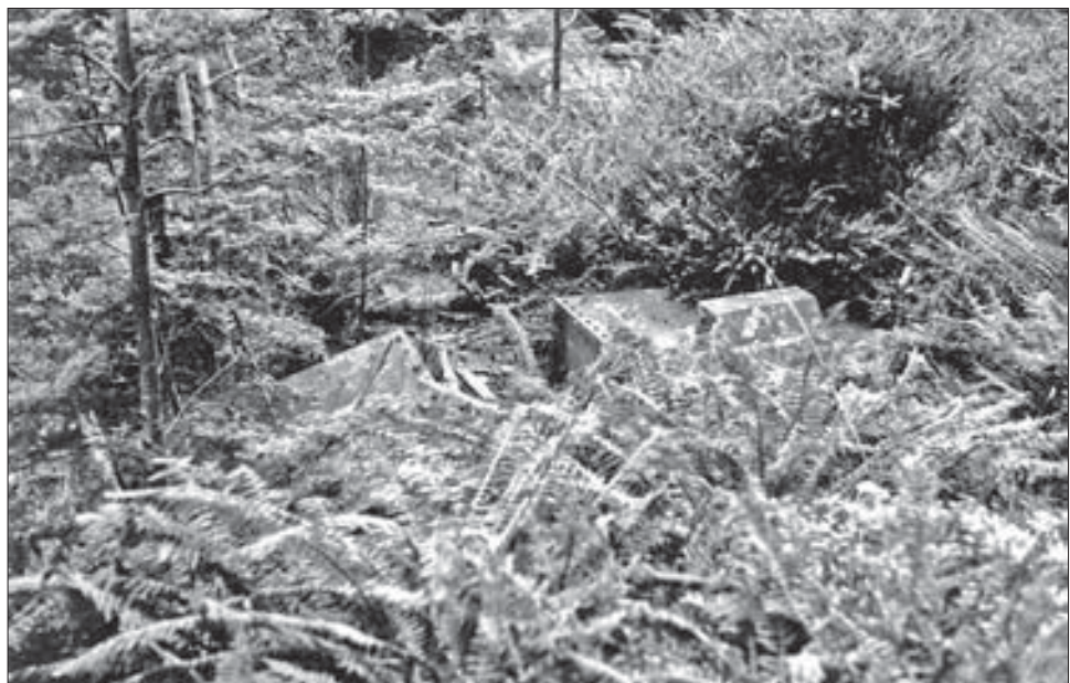
Figure 24. Southberg's Battery, 1996, showing the two remaining mortar boxes on the site. Photo: P. Petchey.
