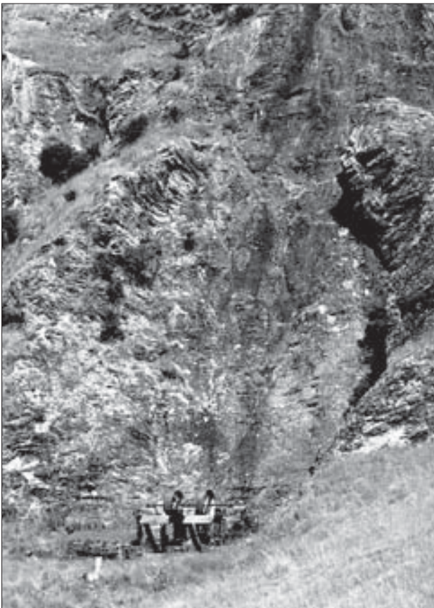
Figure 28. Phoenix dynamos, 1996. The penstocks for the Pelton wheels came down the rock face at the rear of the installation. Some iron supports are still visible in the schist. A similar view to that in Fig. 26.
