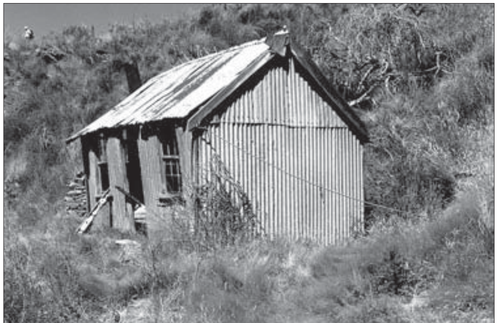
Figure 35. Hut I, Bullendale, prior to restoration in 1998. Photo: P. Petchey.
