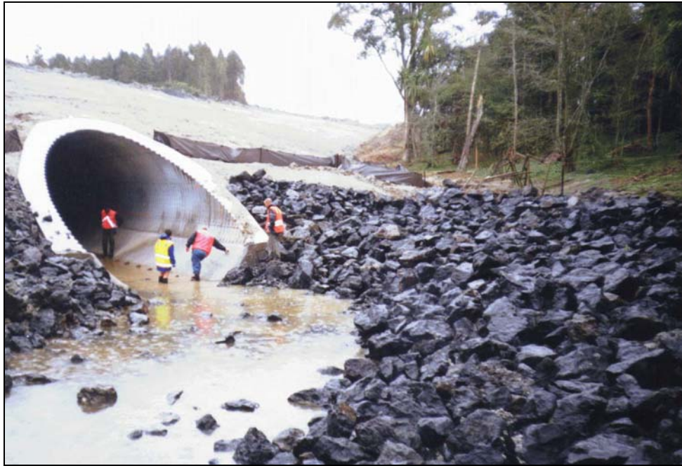
Plate 5. Use of riprap to protect streambed and streambank at the outlet.
