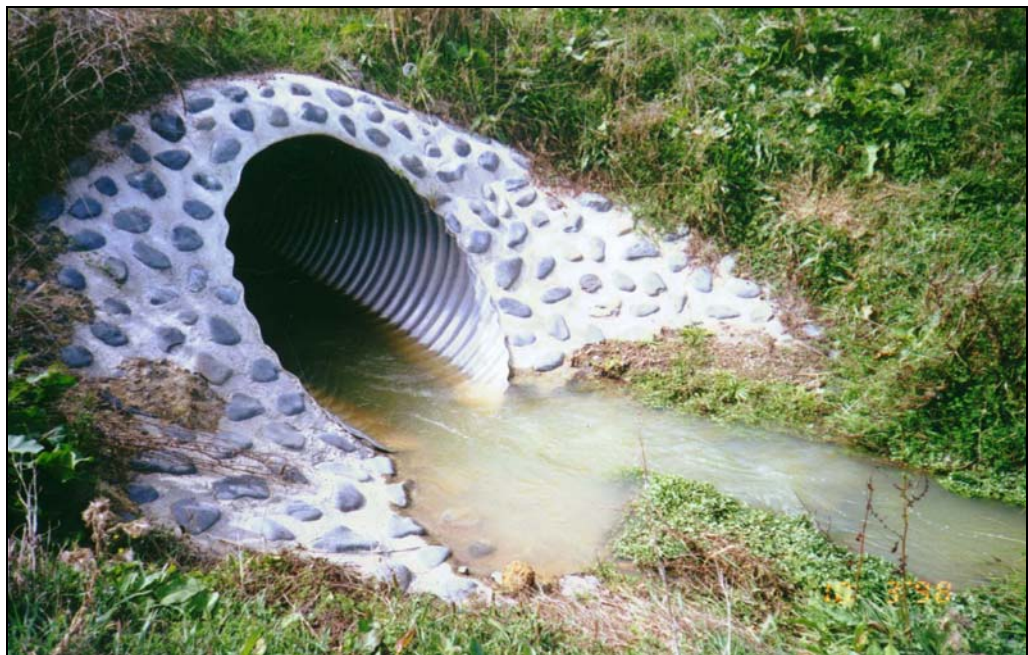
Plate 4. Bevelled culvert inlet. This type of inlet reduces entrance contraction considerably and therefore is less of a problem for fish exiting the culvert. Fish passage in this culvert could have been further improved by using more stones over the culvert end, especially in the lower part of the headwall.
