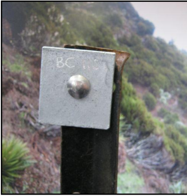
Figure 30. Corner P marker. Waratah with 8 mm stainless cup head bolt with Nylock nut used to attach a 50 × 50 mm square washer.
