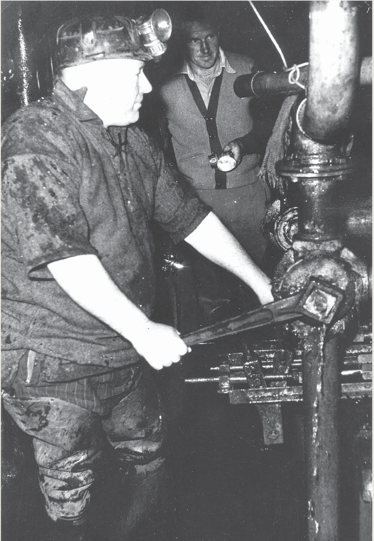
Photo 18: Bob Philp opening the pressure valves on the hydraulic hoist.
