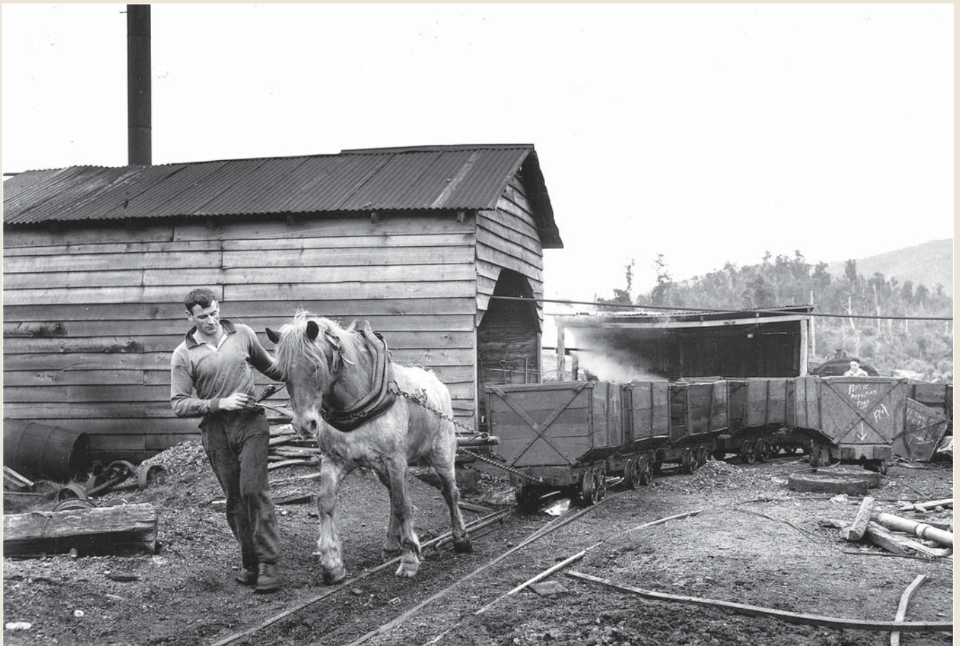
Photo 15: Danny Laurie with Speedy hauling a rake of trucks back to the mine from the bins at the 2nd Mine in 1948. The workshops are on the right, the winch shed is behind the tubs in the middle of the image. NATIONAL PUBLICITY STUDIOS
