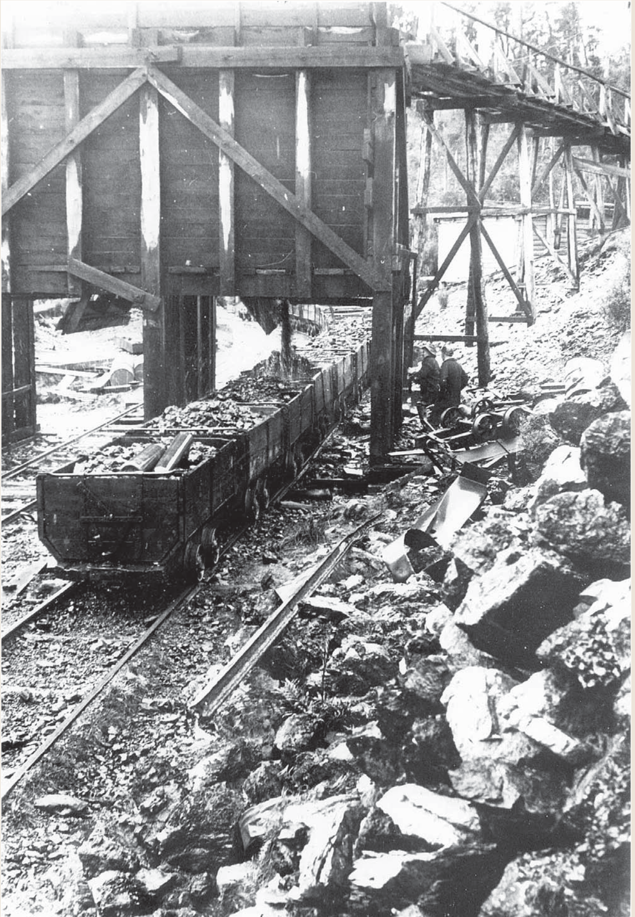
Photo 17: Coal being loaded into trucks from bins at second mine in 1956
