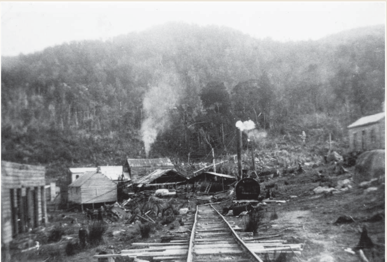
Photo 3: Watson's Mill. The boiler adjacent to the track operated the aerial logging system. The stables are on the far left.
