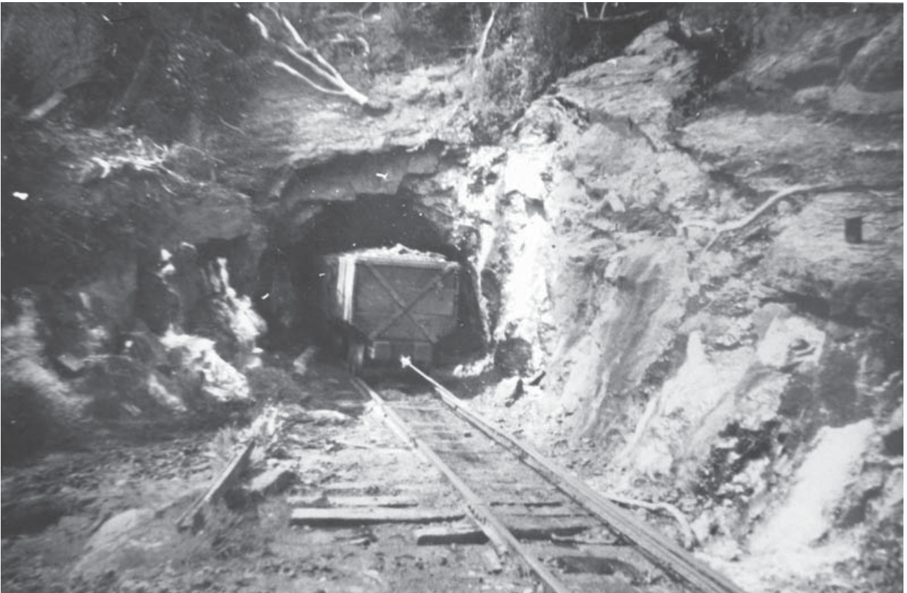
Photo 16: Second mine portal some time after 1943. Note the trucks being hauled out by a winch and wire rope.
