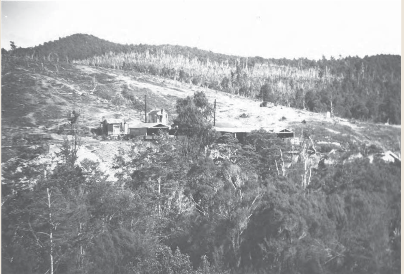
Photo 14: Another view of the second mine site from across Charming Creek. The mine portal is to the left of the image, out of shot. The workshop/blacksmith is obscured behind the tall tree in the centre. The bins are at the right of the complex of buildings.
