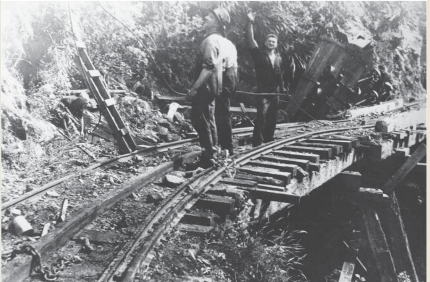
Photo 10: Recovering gear after an accident on the Charming Creek Tramway. A bogey hangs precariously off the edge of the tram, behind the waving figure.
