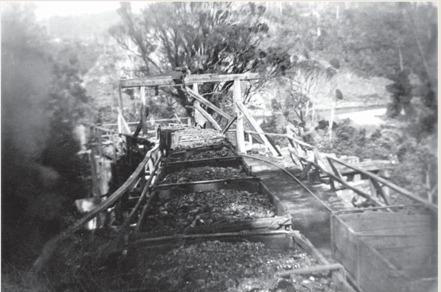
Photo 9: View of the tipper at the top of the Ngakawau bins.
