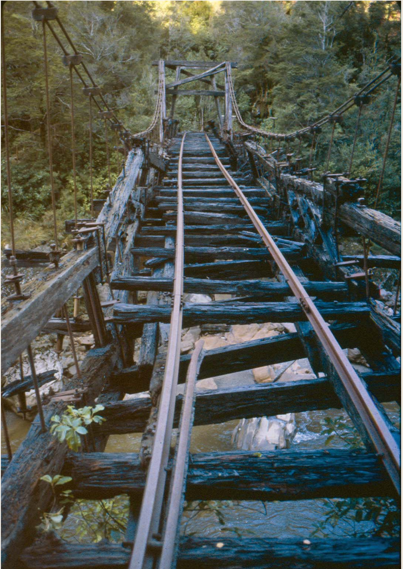
Photo 23: Looking across the bridge over the Ngakawau River, around 1975/76. J. Staton
