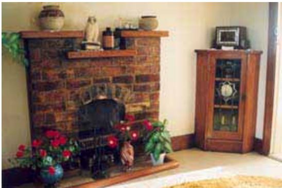
Detail of fireplace, built in tapestry bricks.
