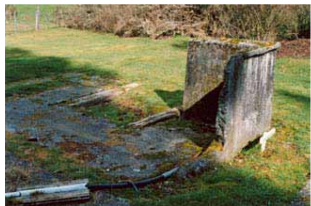
Remains of the original boys' toilet.
