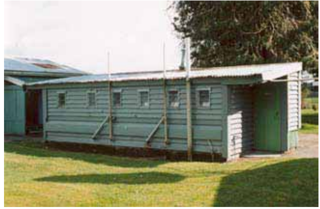
Toilet block, from the east.
