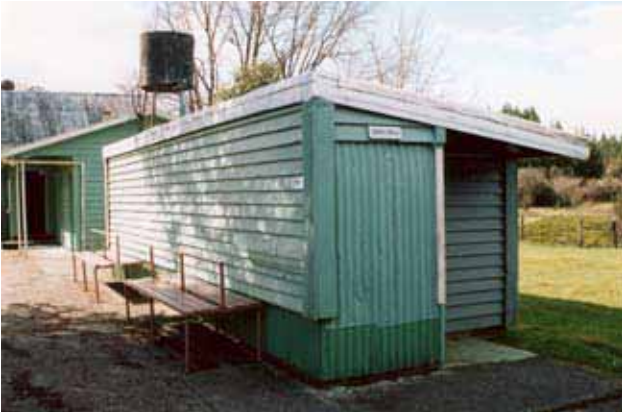
Toilet block, from the south.
