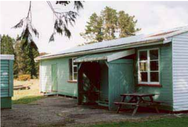
Classroom, north elevation.
