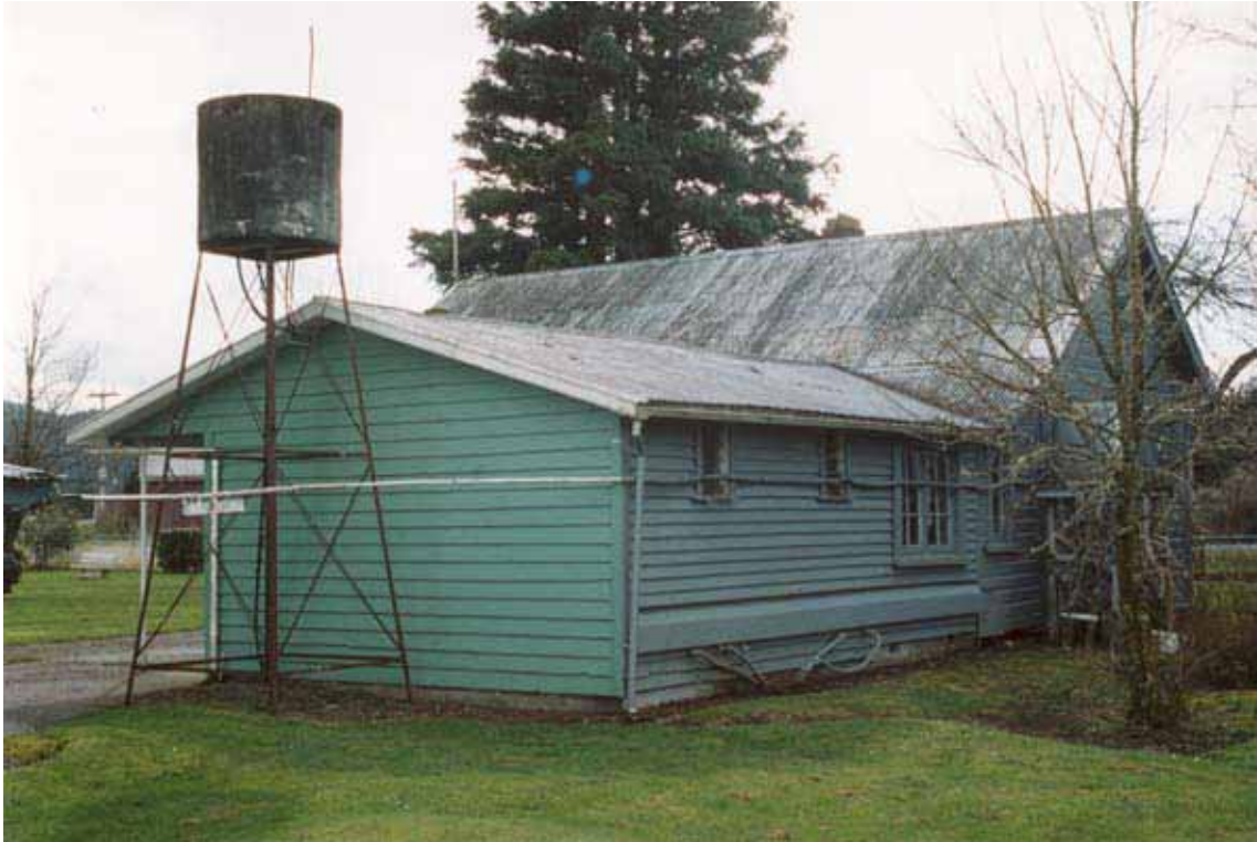
South and east elevations.
