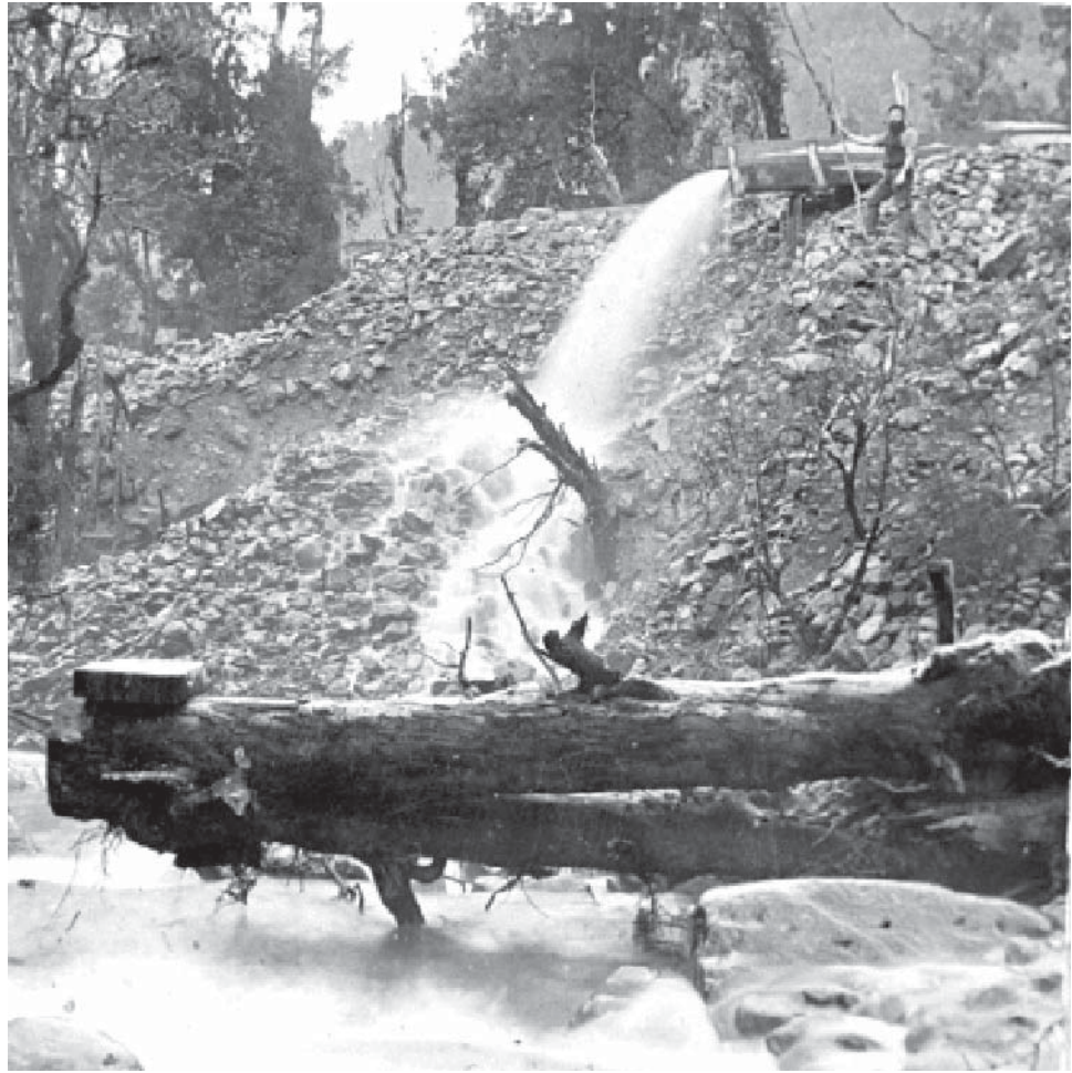
Figure 3: Sluicing Claim at Roaring Meg Creek - workings would have been very similar at Blackball Forks
