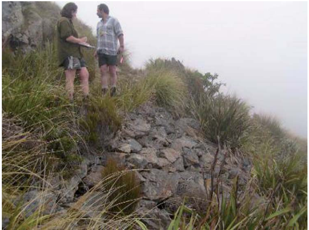
Figure 26: Stacked rock retaining 14
