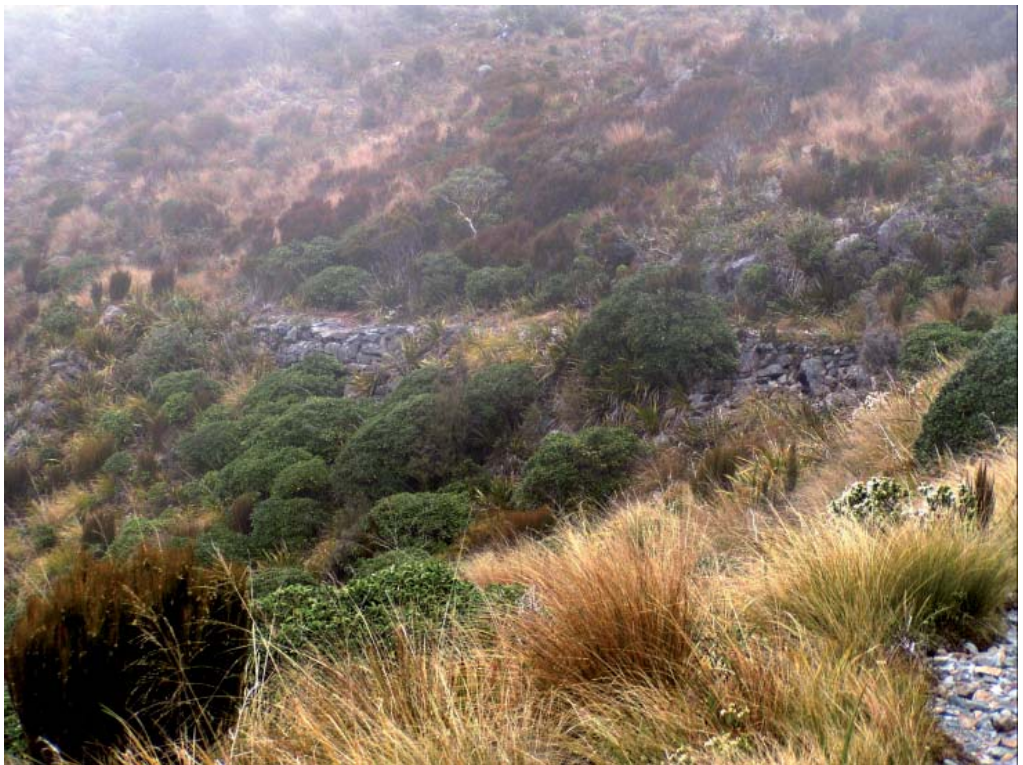
Figure 27: View of long section of rock retaining above Ces Clarke Hut, partially obscured by low vegetation.
