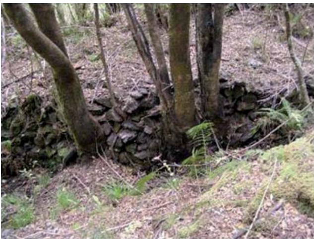
Figure 18: Stone revetting on western end of tail race that goes under track
