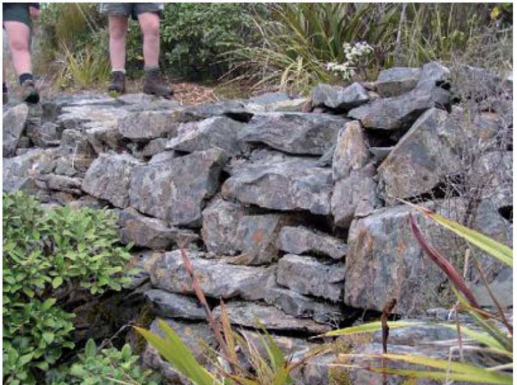
Figure 29: Stacked stone retaining below cut-out 35
