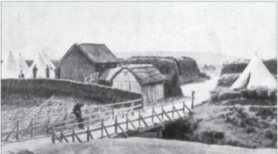
Above: a view of the two-storied Orakau blockhouse, built in 1867. (Cowan collection, Alexander Turnbull Library.) Below: 57th Regiment redoubt beside the Manga-o-hoi Stream, near the intersection of Gorst and Mutu Streets, Te Awamutu.
