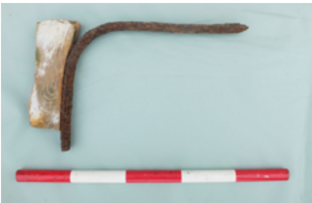
Figure 86. A light rib or stud with an iron bracket attached, 2018. Photo: Peter Petchey.
