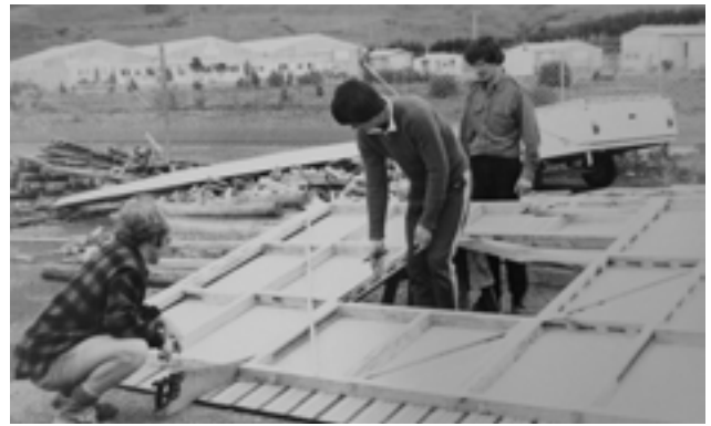
Figure 18. Cutting up the BAAS hut into units for transportation at Tūrangi in 1978. Photo: Newton 1979; Archives New Zealand Te Rua Mahara o te Kawanatanga, Dunedin Regional Office.
