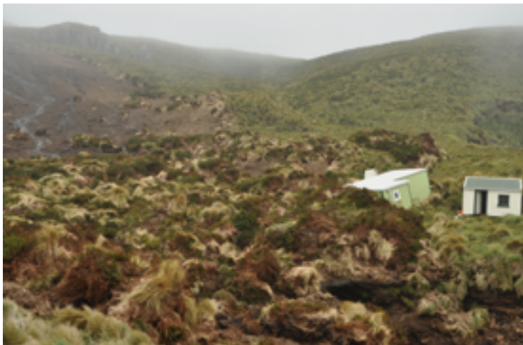
Figure 23. The aftermath of the 2014 landslip, with the 1978 BAAS hut pushed towards the castaway depot hut, 2014. Photo: Kath Walker.
