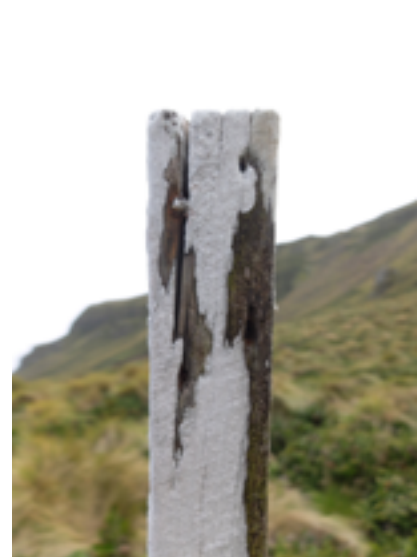
Figure 151. The top of the South Bay fingerpost (2018), showing the white lichen and nail holes where the fingerboard was attached. Photo: Peter Petchey.
