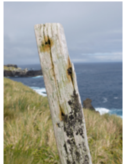
Figure 144. The top of the south coast fingerpost (2018) showing the nail holes where the fingerboard was attached. Photo: Peter Petchey.
