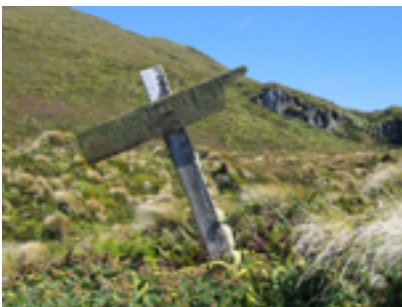
Figure 126. The Alert Bay fingerpost in January 2004. The light angle shows that the lettering stands proud of the rest of the board: this is due to the paint of the letters providing some protection from weathering for the underlying timber. Photo: Kath Walker.
