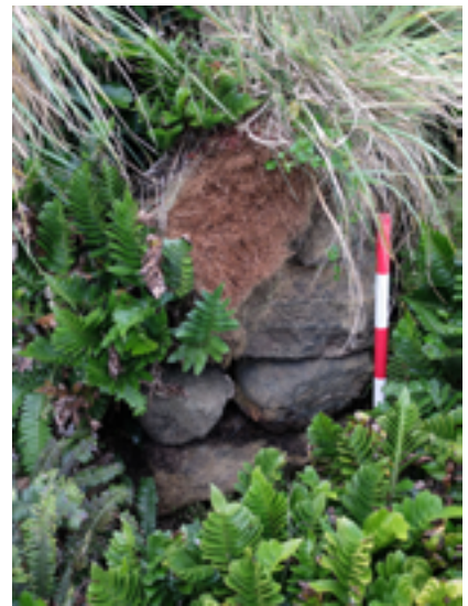
Figure 112. The stonework of Hut 3 (0.5m scale in 100mm units), 2018. Photo: Peter Petchey.
