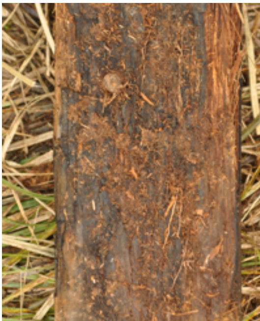
Figure 76. Close-up of the timber lintel showing one of several tacks which may have held sailcloth to it to shelter the fire from rain, 2015. Photo: Kath Walker.
