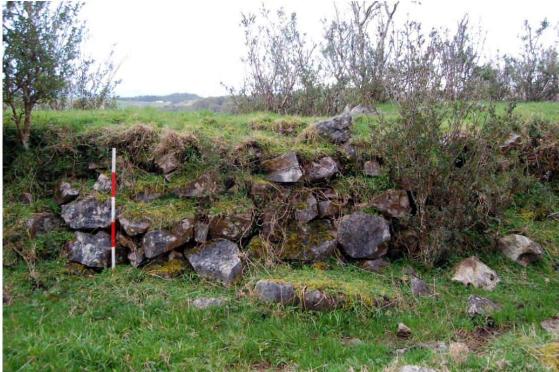
Figure 3: Close-up of a section of the tramline, showing the rough construction of the stone facing
