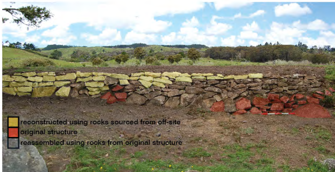
Figure 6: The repaired section of stone facing
