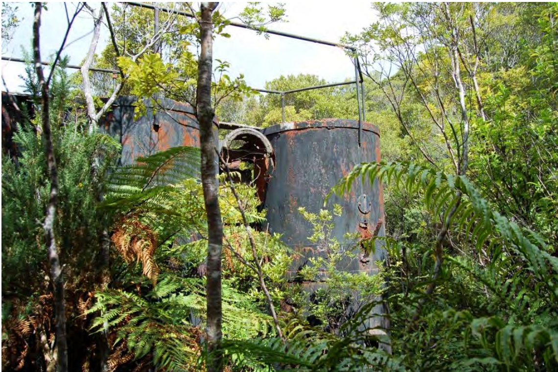
Figure 7: Towers. Above: Southern aspect of towers in 1968. Note handrail around the top and large inlet pipes connected to the “exchange” by way of terracotta pipes. Photo from the collection of Anne and Brian Reed. Below: Northern aspect of towers inn April 2010. Note the large “outlet” pipe.
