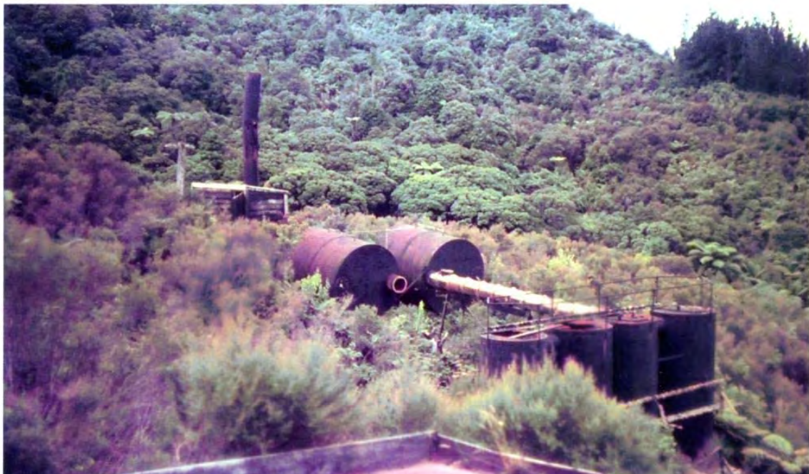
Figure 6: Above: Looking east across the lake in 1968; the dam is in the middle ground, and the roads flanking the lake are clearly visible (see figure 3). Below: Looking north at the towers (bottom right), the tanks, and the building which housed the fan/exhauster.
