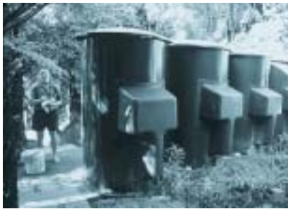
DoC probably maintains more toilets than anyone except the nation's schools. These are in Abel Tasman National Park. Andy Dennis
