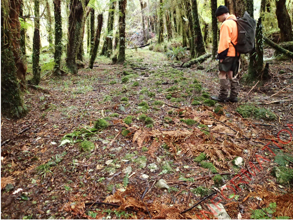
Figure 14. A long section of intact cobbled track surface. This section, recorded as WP 106, is approximately 2 m wide and extends approximately 25 m along the track. There is cut drain along the upslope (right) side of the track.
