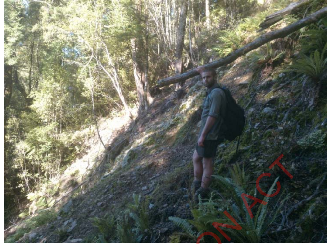
Figure 10: There are a number of small slips in the lower Pike Valley. Potential erosion issues exist but these will be easy to manage with sympathetic track profile setup and execution.
