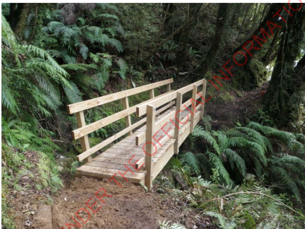
Figure 5: Typical bridge over small water course
