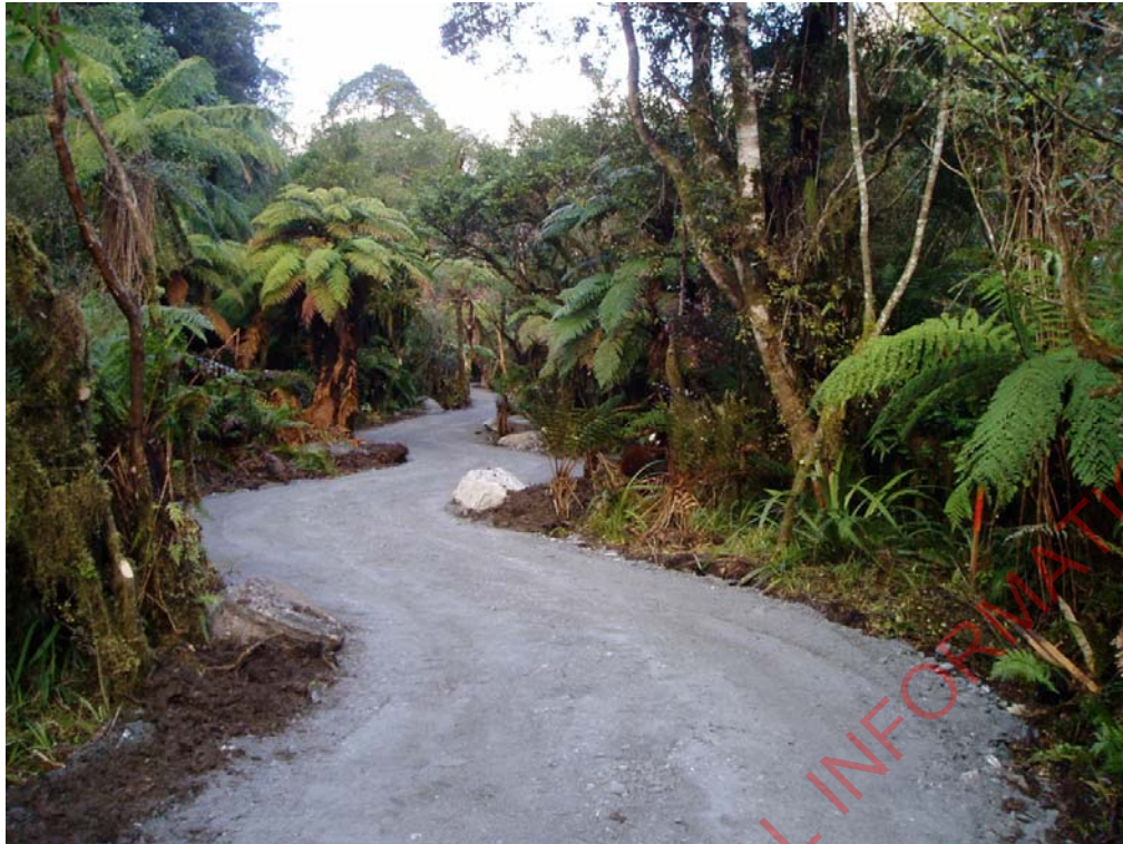
Figure 12: Stage Three - Placement of organic matter and topsoil along path verges.
