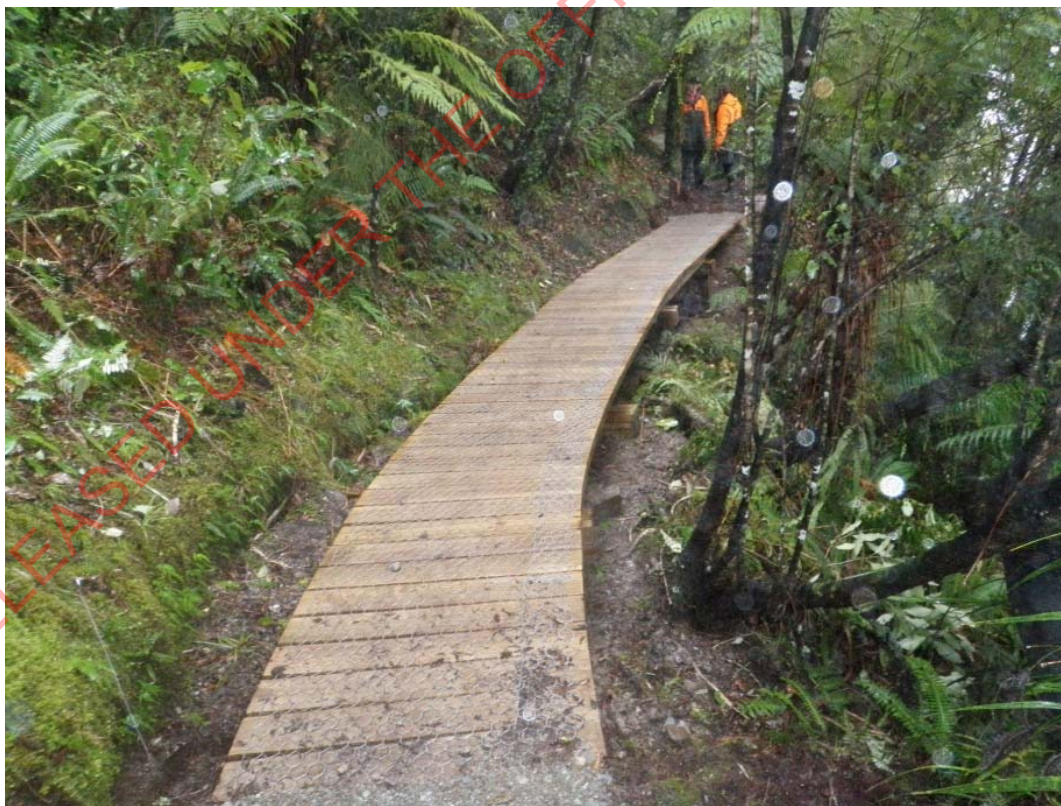
Figure 8: Boardwalk as constructed through a forested landscape.
