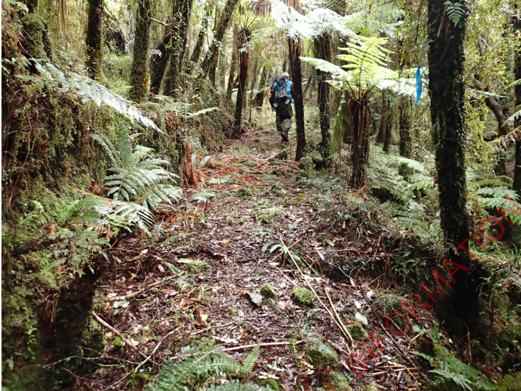
Figure 13. A section of benched track.
