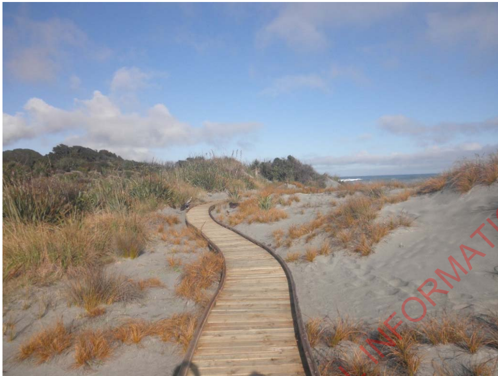
Figure 7: Completed boardwalk at Ship Creek Track.
