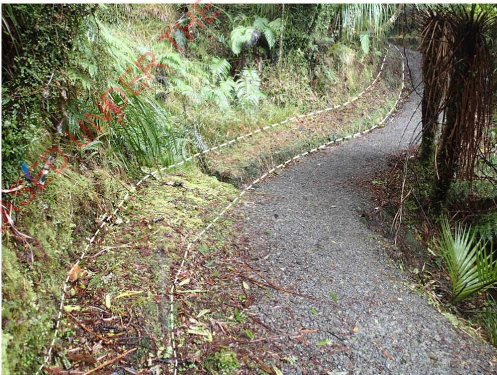
Figure 9. A typical section of track with the original track surface on the upper bench (white lines) with the more modern track running beside it.
