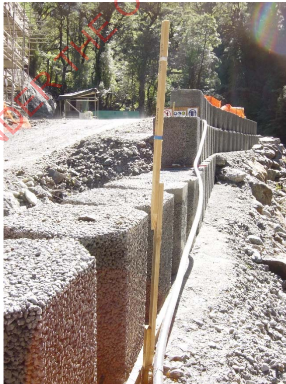
Armour works being installed above White Knight Stream
