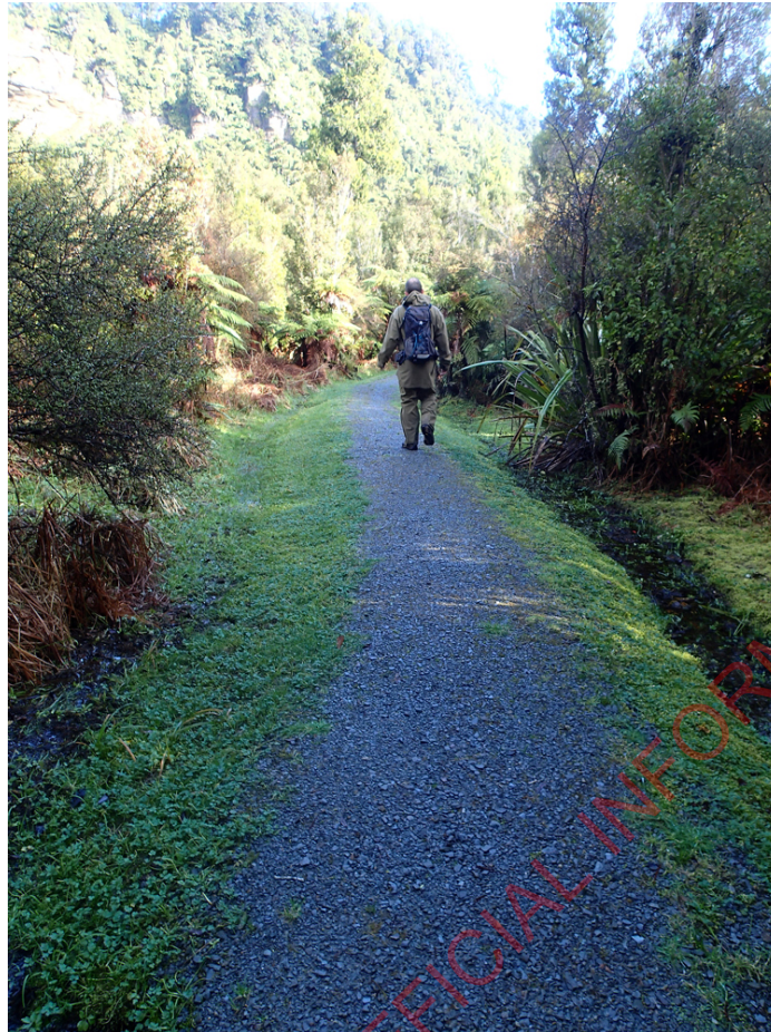
Figure 7. A section of the lower track, near the Punakaiki River, showing the original raised track with drains on either side.
