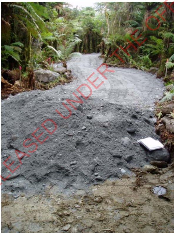
Figure 11: Stage Two - Stripping of organic matter and topsoil to stockpile for later use, and placement of basecourse.
