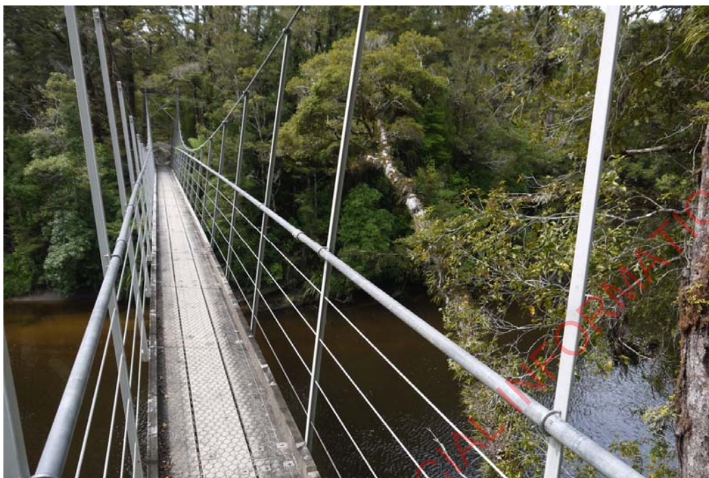
Figure 4: Typical suspension bridge
