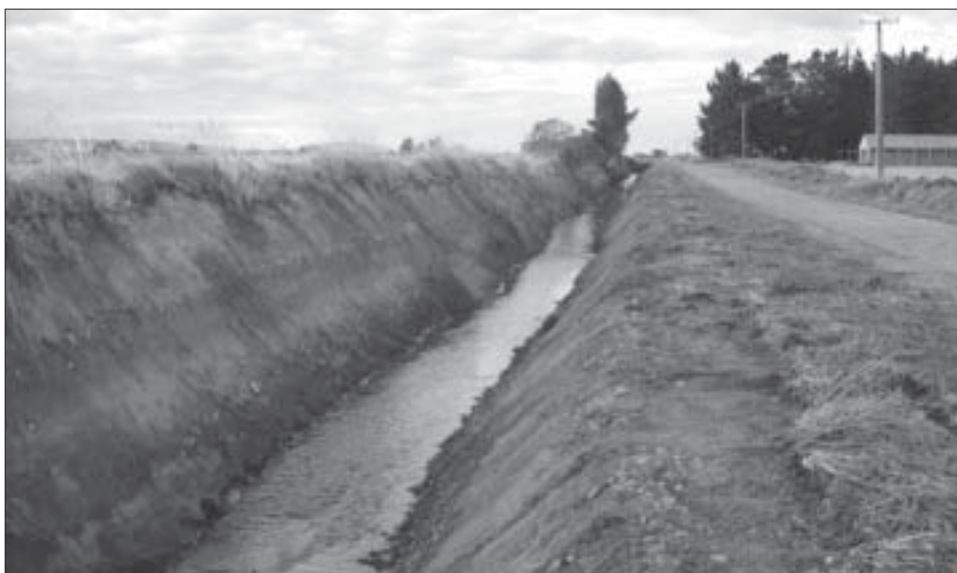
Figure 5. A roadside drain from which all in-stream and riparian vegetation has been removed, leaving no habitat for aquatic wildlife and biota.
