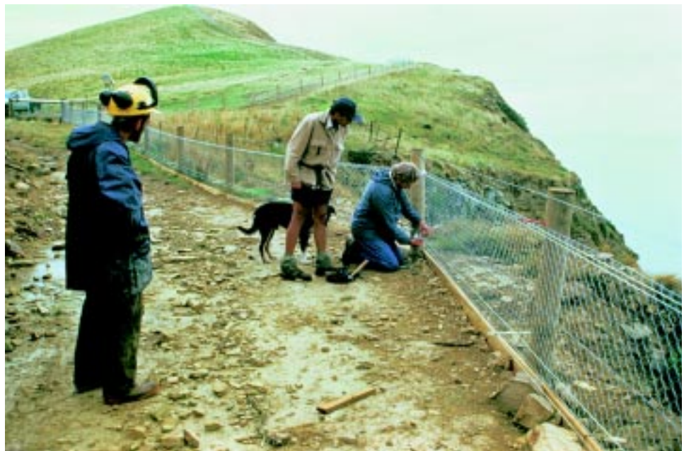
Fence construction at Cape Lambert. (DOC)
