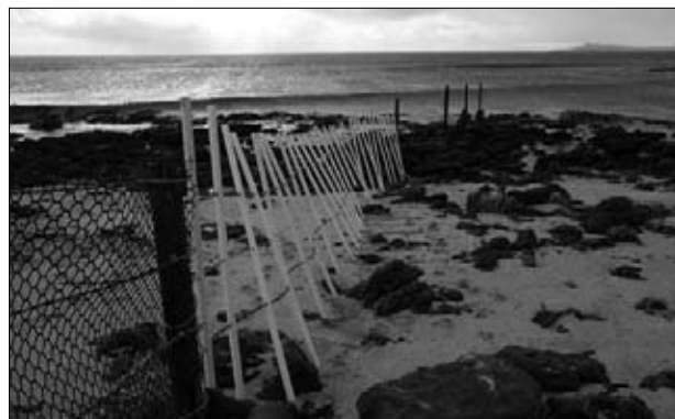
Figure 14. A fence tie-off extension of plastic poles designed to prevent stock entering Tioriori. Part of the original version of steel waratahs, wire cables and plastic mesh is visible to the left of the photograph, and concreted onto tidal rocks in the background. Photo: Peter Moore.
