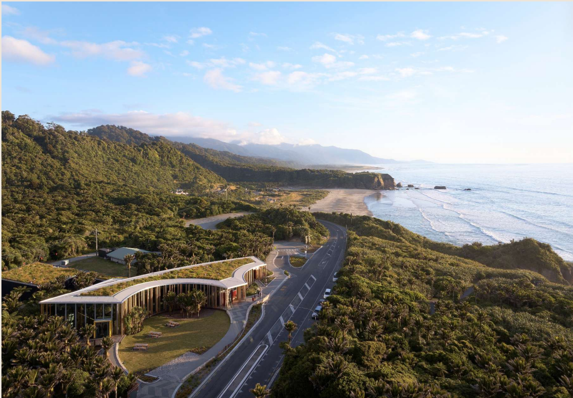
Punangairi Visitors Centre, Dolomite Point. Source: Ngāti Waewae and Department of Conservation
