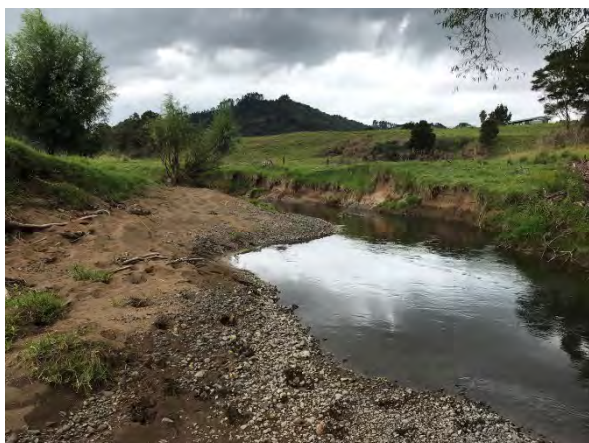
Photo 10: Erosion of material on inside of point bar and slumping. Erosion is likely to have been exacerbated by stock access.
