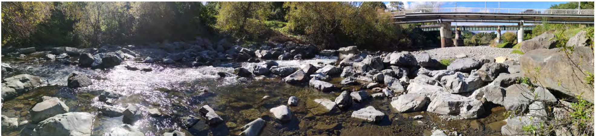
Figure 2-10 (A) The weir below the SH1 and rail bridges in November 1979, then a concrete-block structure; it was replaced by the present rock weir in 1985 (Crown aerial photograph 5614 F 27). (B) The heavy rock ballast of the weir, looking upstream, April 2022.
