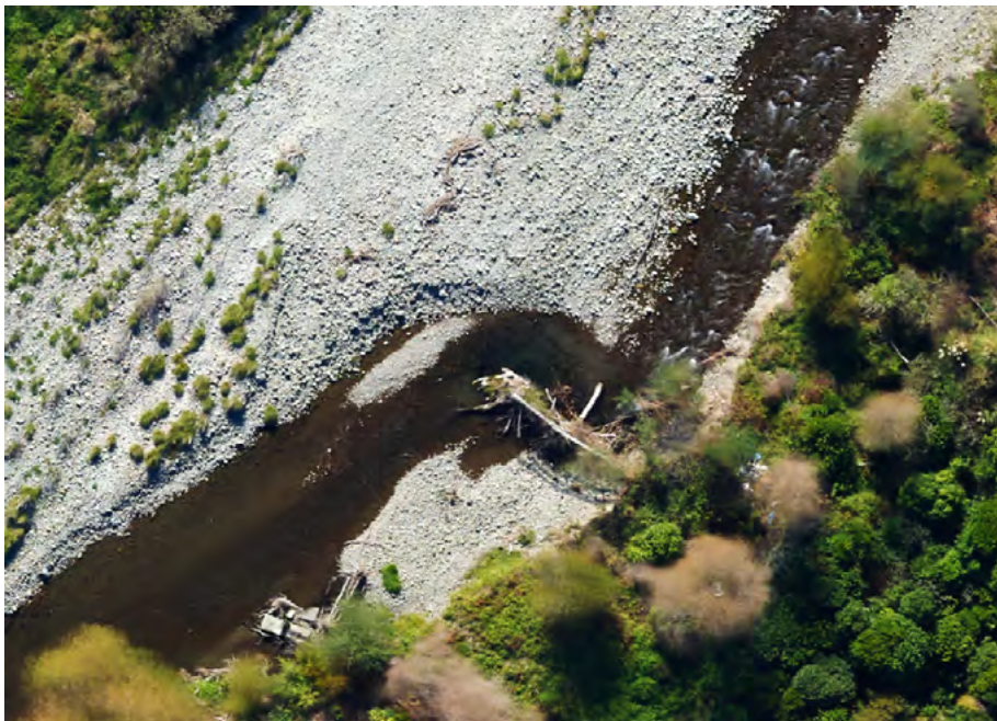
Figure 4-7 Forced morphologies. (A) Three rock groynes near XS 345 anchor pool formation. (B) Woody debris near XS 390 has caused local scour and deposition on the right bank.
