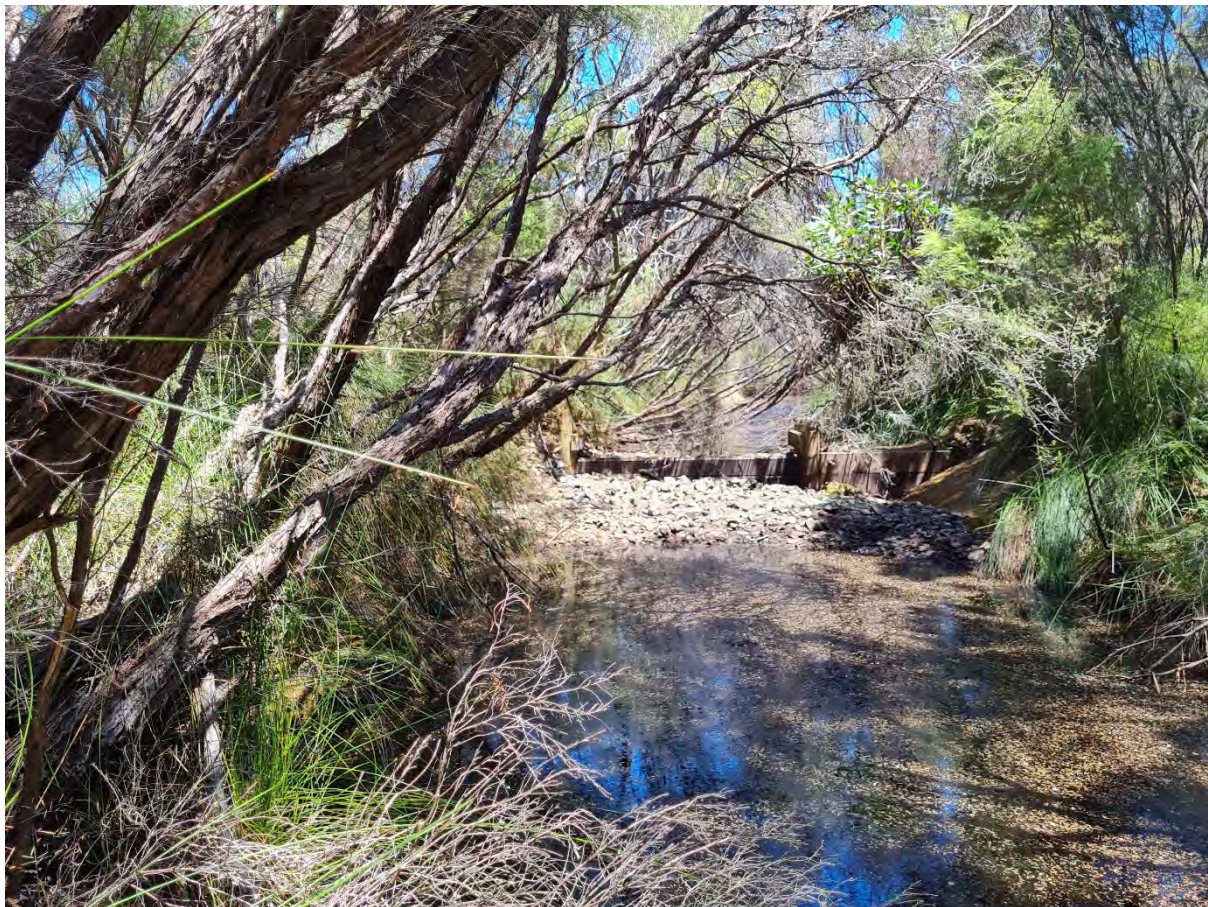
Figure 11. View looking upstream at the existing weir which is currently poorly functioning and could be upgraded to improve the hydrology of Lake Ohia.
