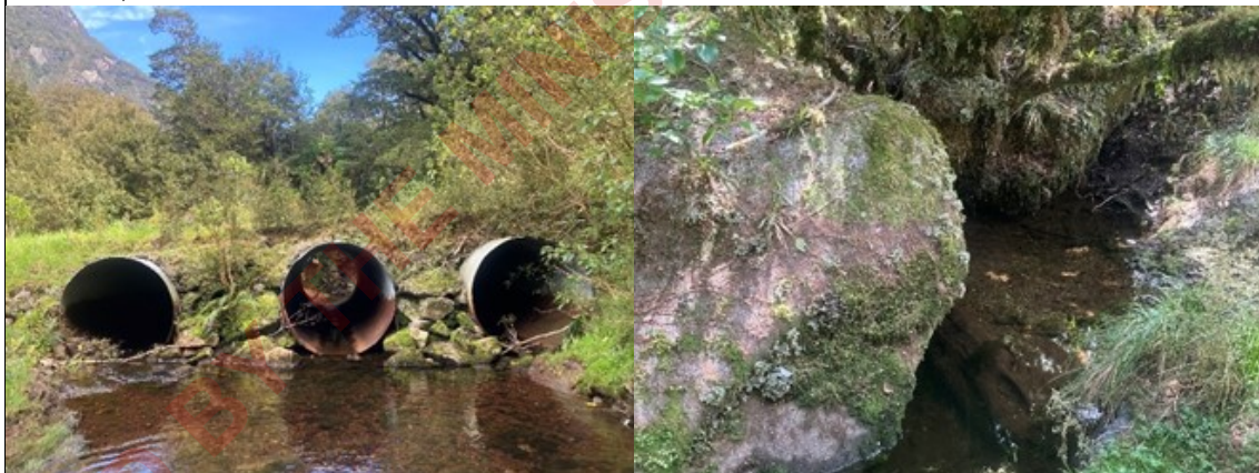
The multi-barrel culvert crossing at Tarn Creek, Little Tahiti. An isolated pond, where galaxiids were noted, next to the Fish passage is partly impeded through the left barrel, but the middle and right barrel act as a full barrier to fish.
