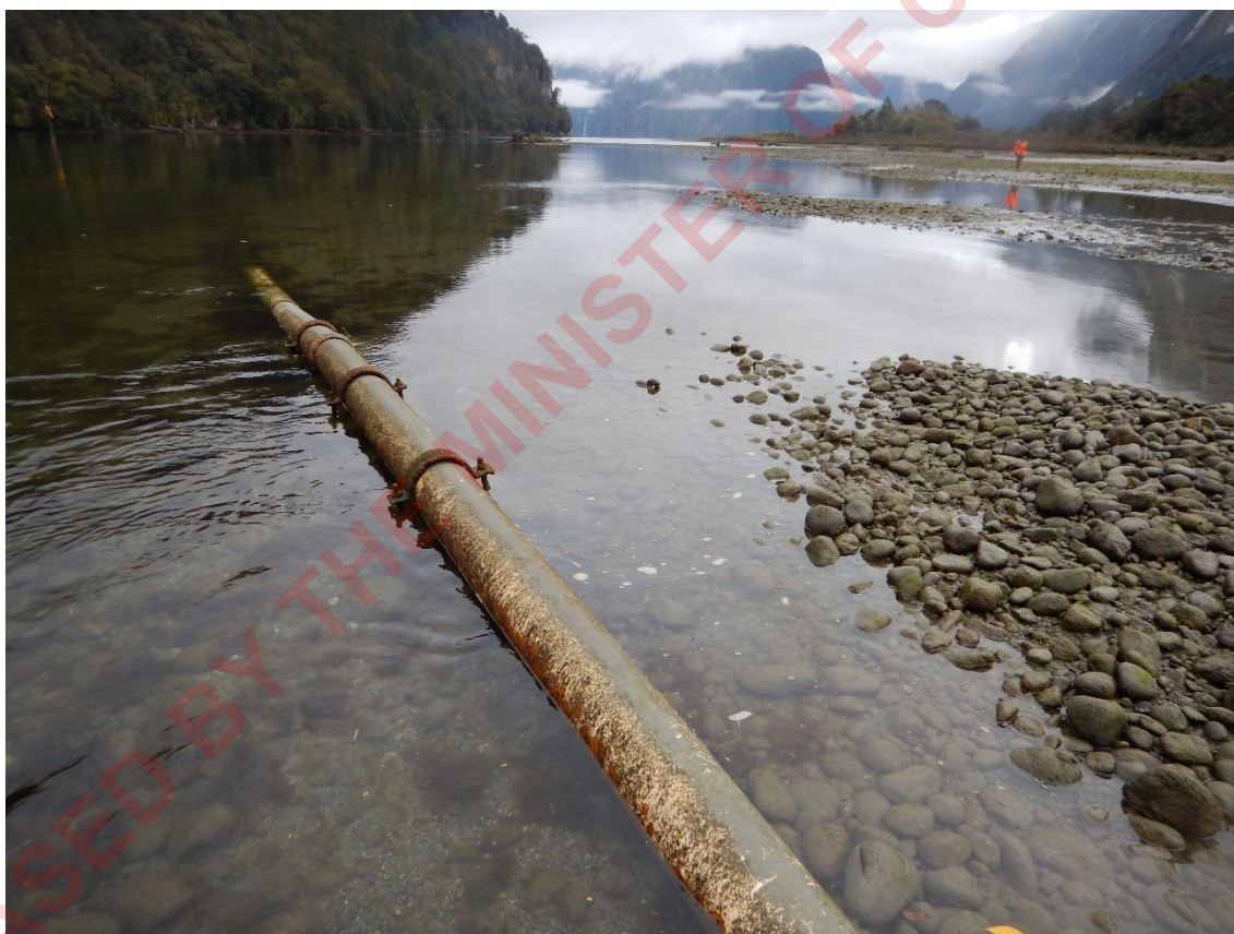
Figure 46. Existing wastewater treatment outfall pipe.
