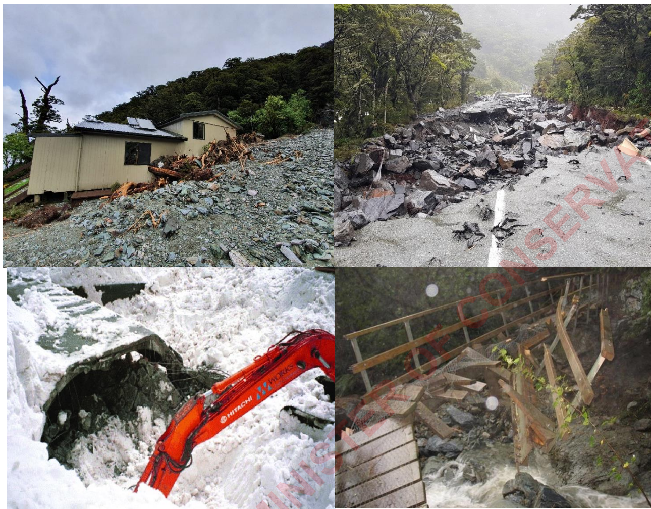
Figure 4: Hazards within the study area. Top left: Rock avalanche/landslide damage to Lake Howden Hut following a storm (source: Luke Bovill – Department of Conservation). Top right: Scouring of the Milford Road due to flooding (source: Dylan O'Neill/Waka Kotahi). Bottom left: The eastern portal of the Homer tunnel damaged by an avalanche (source: Conway et al. 2000). Bottom right: A damaged bridge on the Routeburn track due to flooding (source: Department of Conservation).
