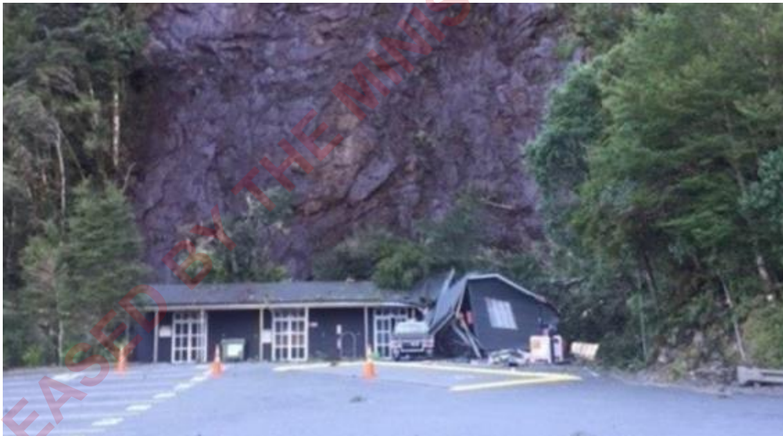
Figure 15: Damage to a storage building in Milford Sound from a rockfall in 2016 (source: Tim Holland).
