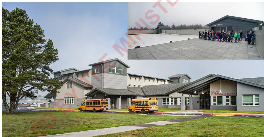
The first tsunami vertical structure in the United States: Ocosta Elementary School, Westport, Washington. The building is designed to withstand an earthquake and has a flat roof over the gym to accommodate up to 1,000 students and community members from a resulting tsunami. Source: Pete Eckert, Eckert & Eckert Photography Download Image
