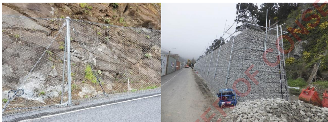
Figure 16: Examples of rockfall and landslide mitigation. Left: A rockfall catch fence in Kaikoura. Source: Geofabrics. Right: A rockfall bund along a road. Source: NZGS
