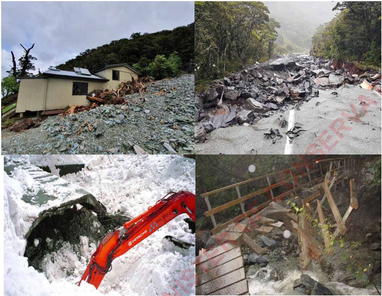
Figure 7: Hazards within the study area. Top left: Rock avalanche/landslide damage to Lake Howden Hut following a storm (source: Luke Bovill – Department of Conservation). Top right: Scouring of the Milford Road due to flooding (source: Dylan O'Neill/Waka Kotahi). Bottom left: The eastern portal of the Homer tunnel damaged by an avalanche (source: Conway et al. 2000). Bottom right: A damaged bridge on the Routeburn track due to flooding (source: Department of Conservation).
