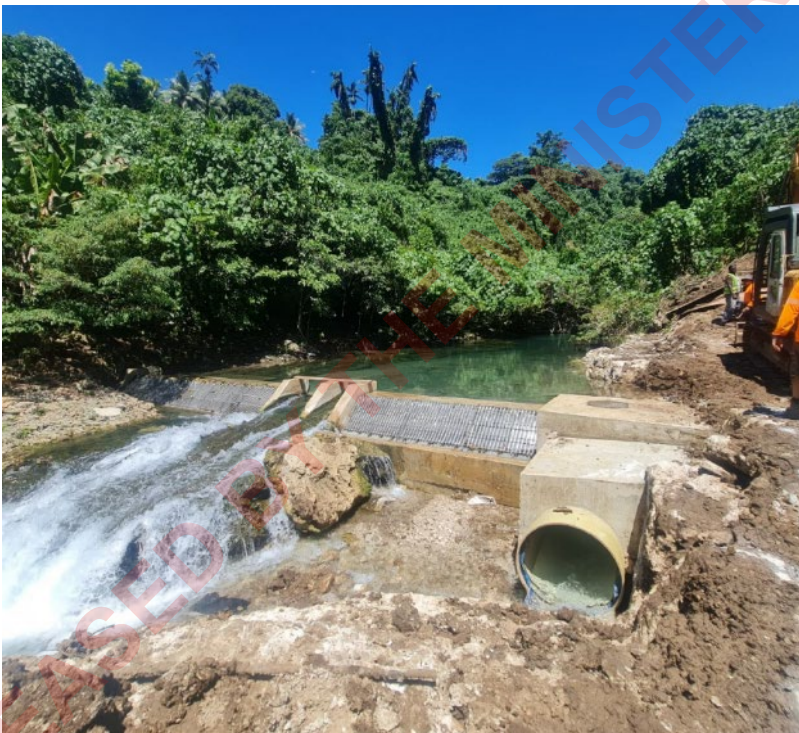
Figure 7-1: Example of small-scale hydropower plant weir and intake works
