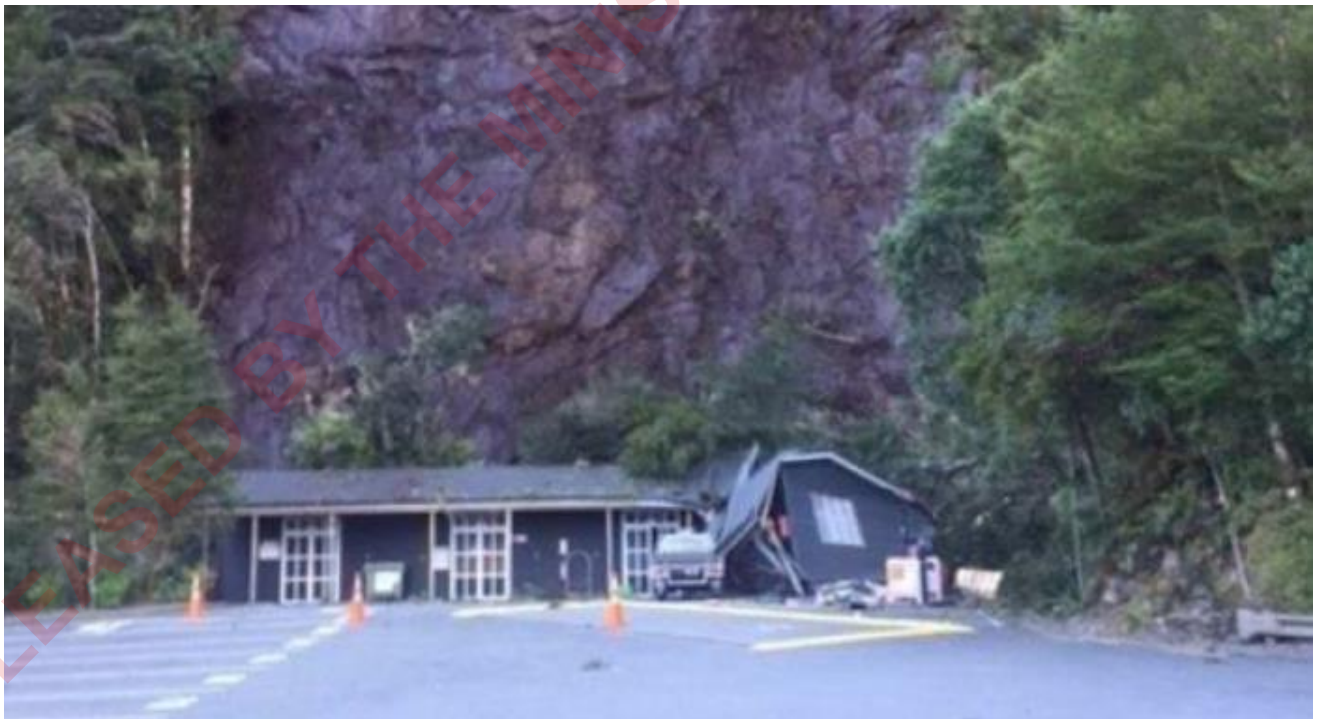
Figure 72: Damage to a storage building in Milford Sound from a rockfall in 2016 (source: Tim Holland)
