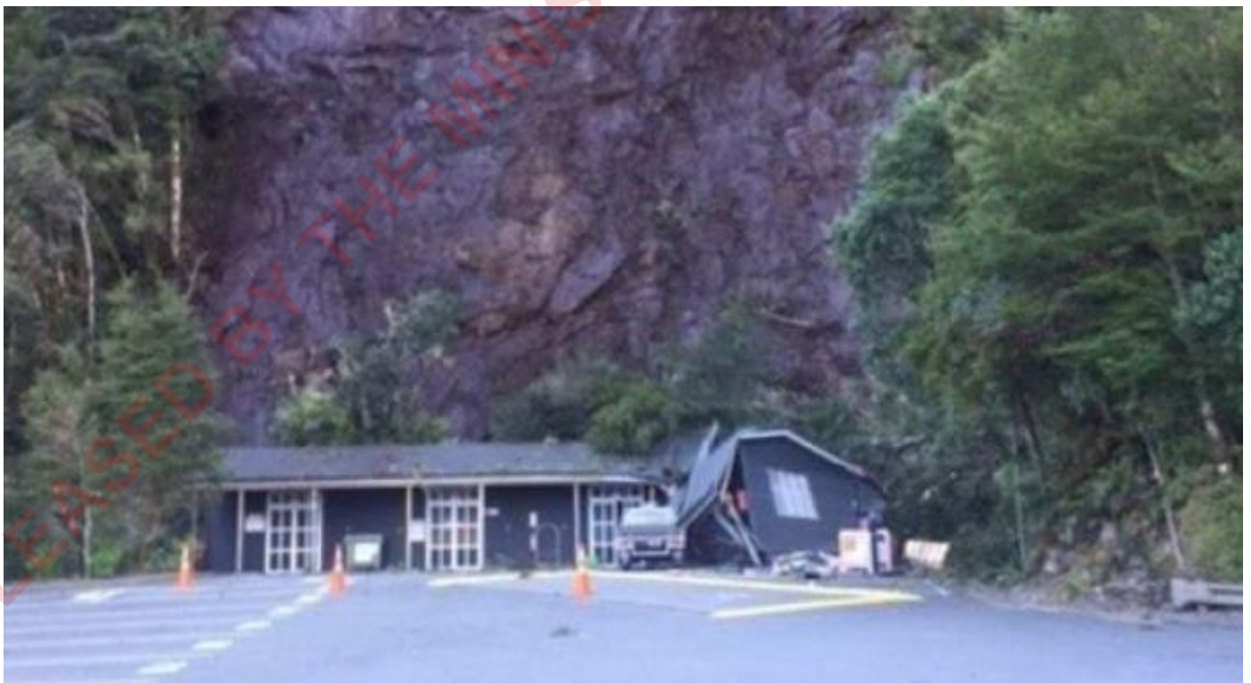
Figure 41: Damage to a storage building in Milford Sound from a rockfall in 2016 (source: Tim Holland)
