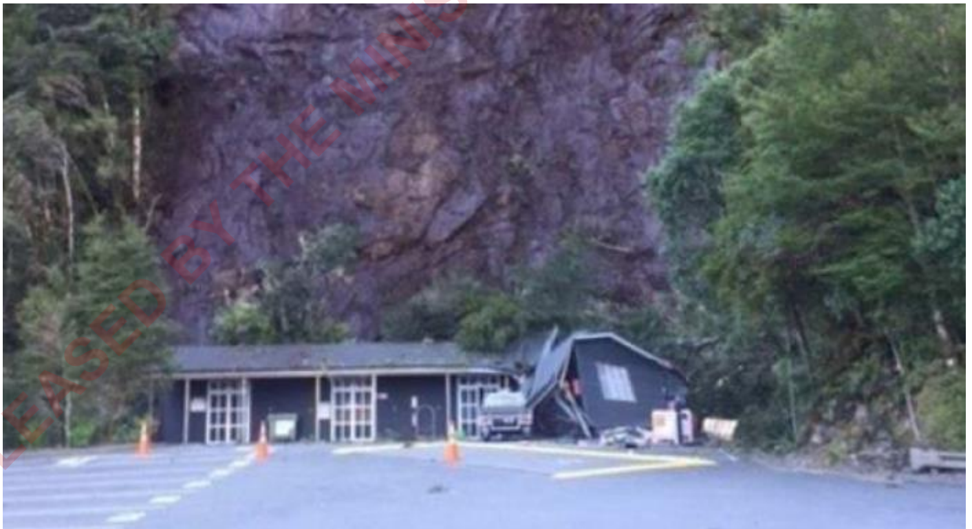
Figure 51: Damage to a storage building in Milford Sound from a rockfall in 2016 (source: Tim Holland)
