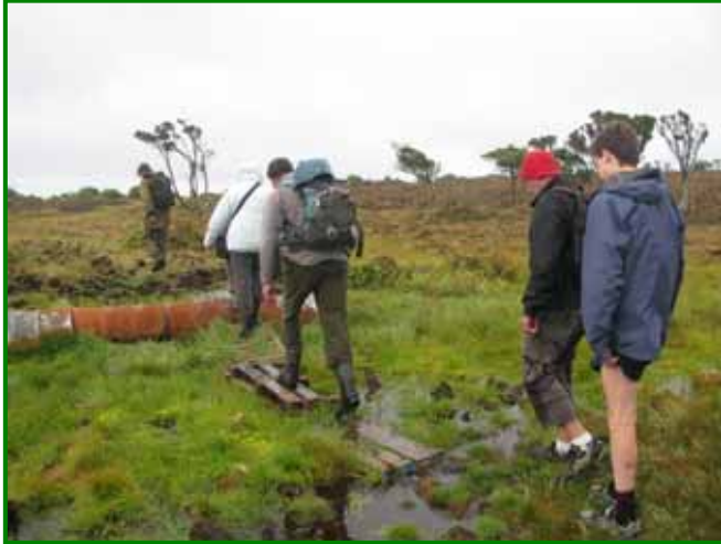
The bridge that DOC Visitor Asset staff erected one month later to replace the pellets and drums pictured in photo on the left
