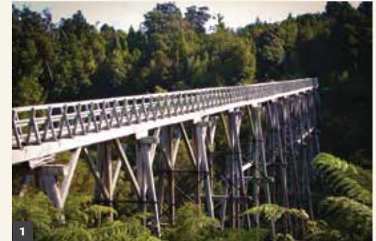
1. The wooden trestle viaduct across the Percy Burn is the largest of four built by the Marlborough Timber Company in the 1920s as part of its logging tramway to Port Craig. The bridges all lie within the West Rowallan SILNA lands and are protected as historic heritage, but the Percy Burn viaduct is currently closed and awaiting restoration. PHOTO: LES MOLLOY
