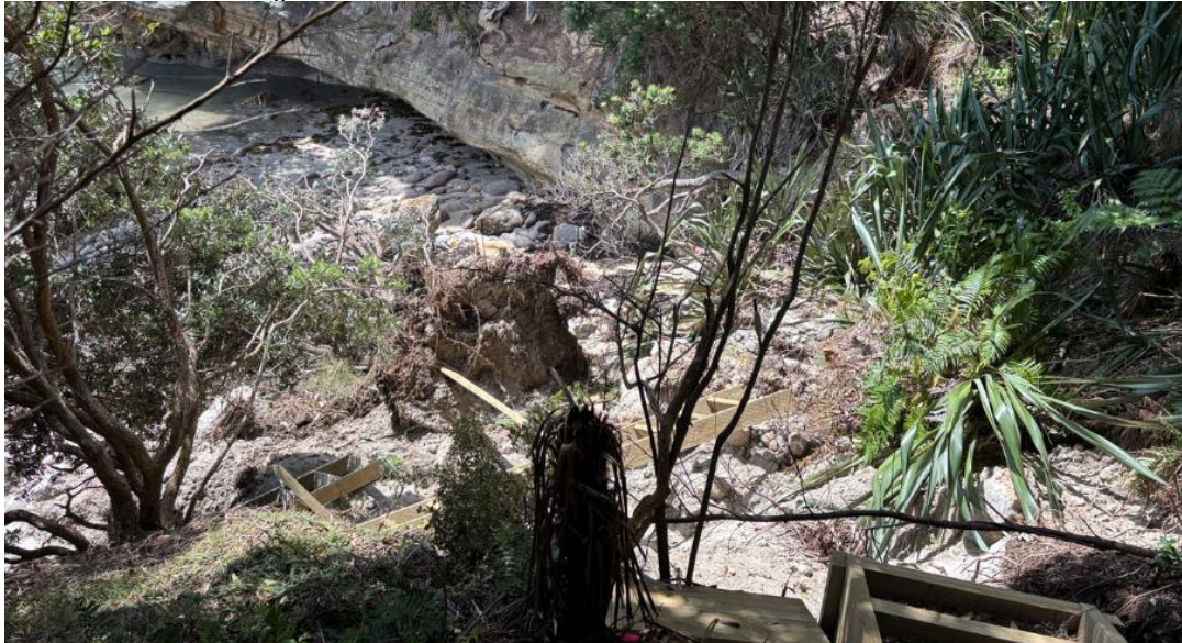
Landslide and track damage: Photo DOC
