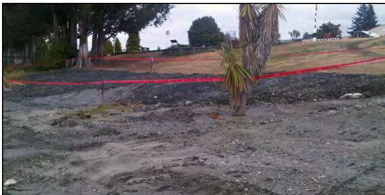
Figure 56 - Photo of the lakeshore after the excavation was completed
