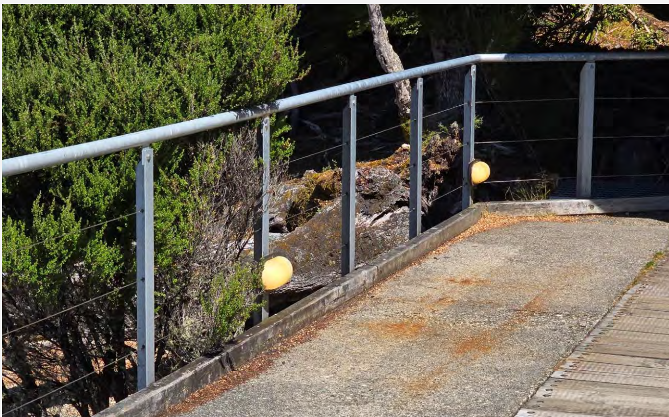
Figure 32 – photo of the type of lighting on Te Ana-au Glowworm Caves wharf
