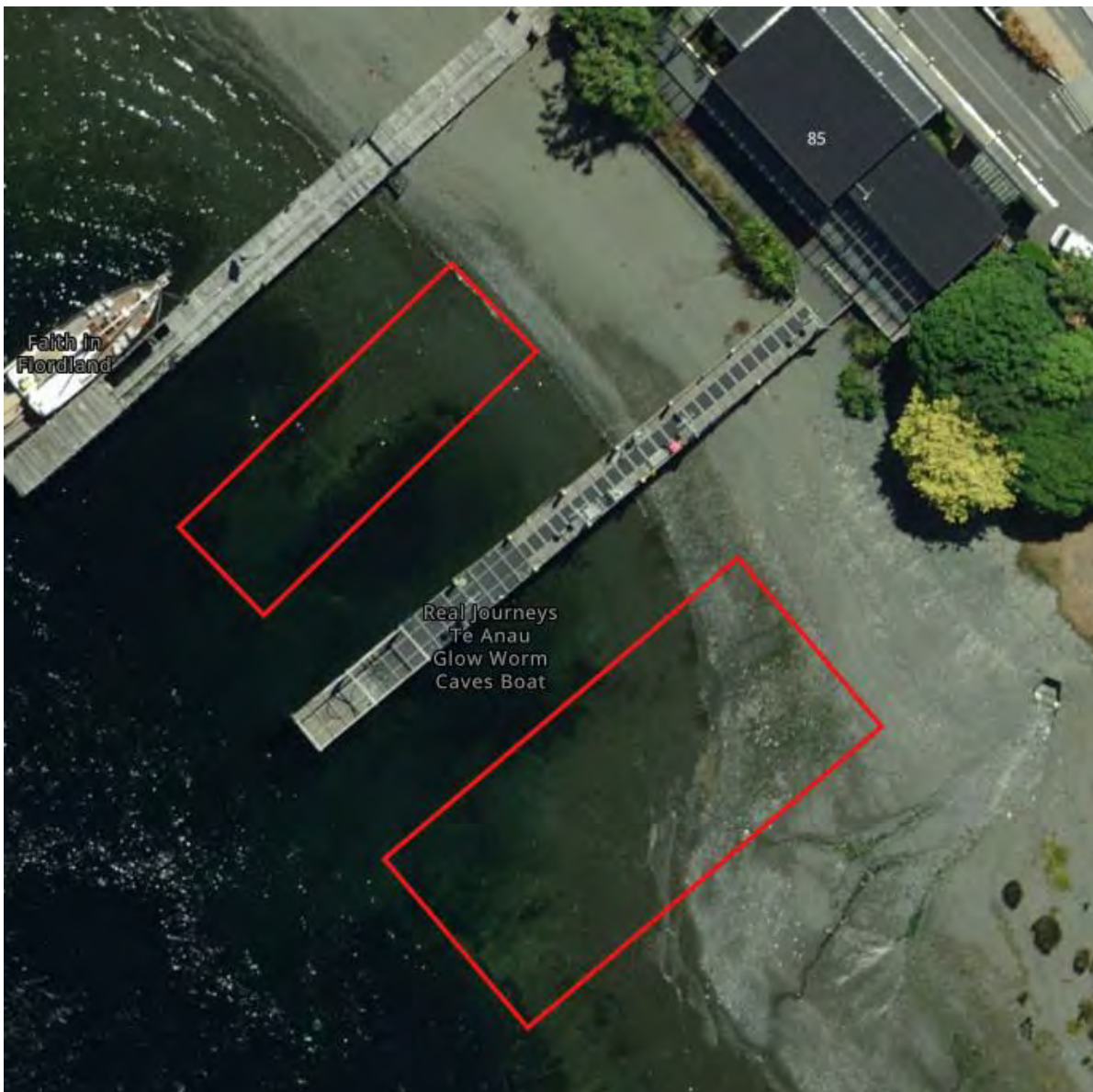
Figure 54 – area photo showing shallow areas in the lake that are likely to require excavation in the future.
