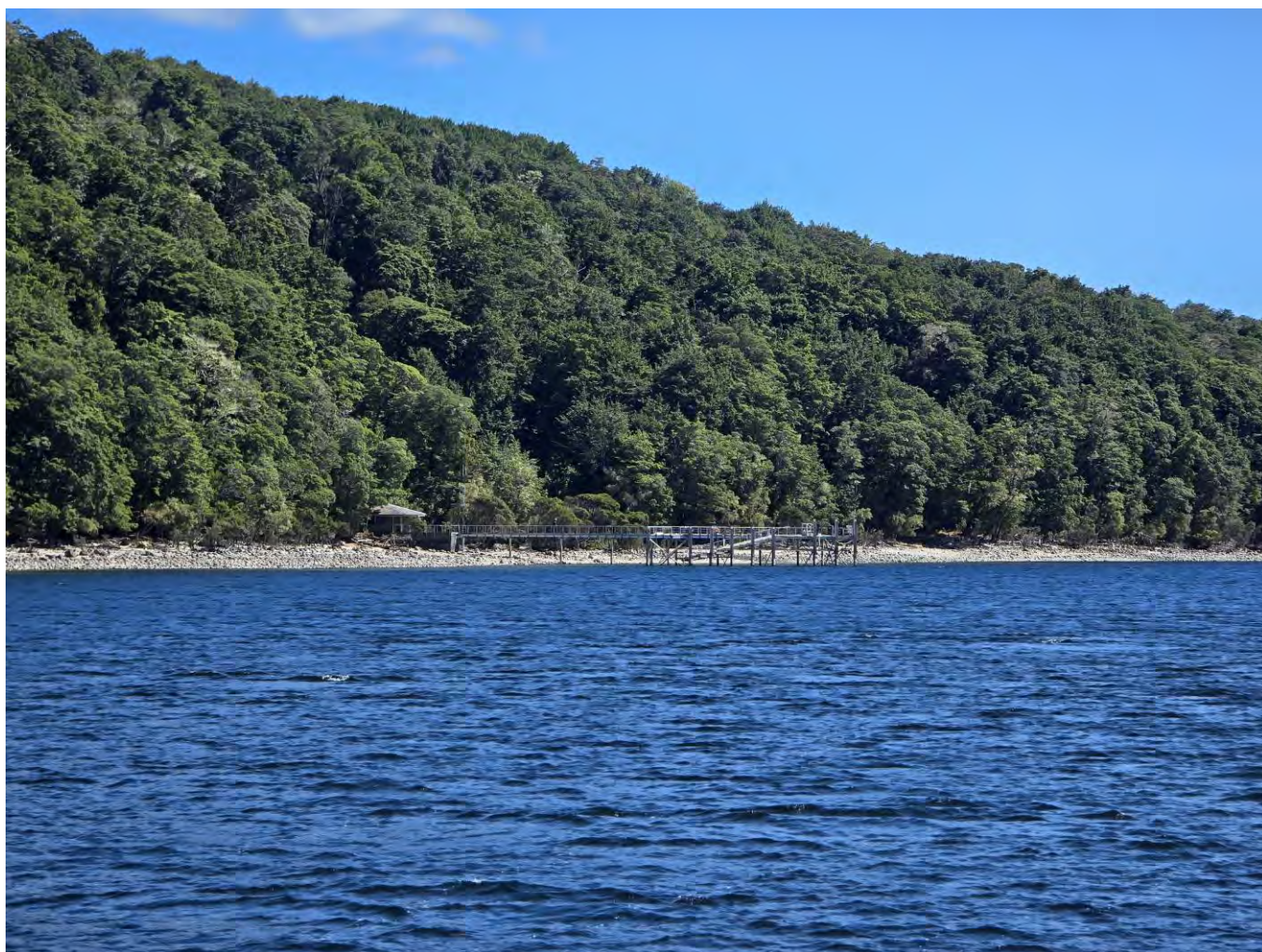
Figure 49 – photo of the Te ana-au Glowworm Caves Wharf when approaching from the south.
