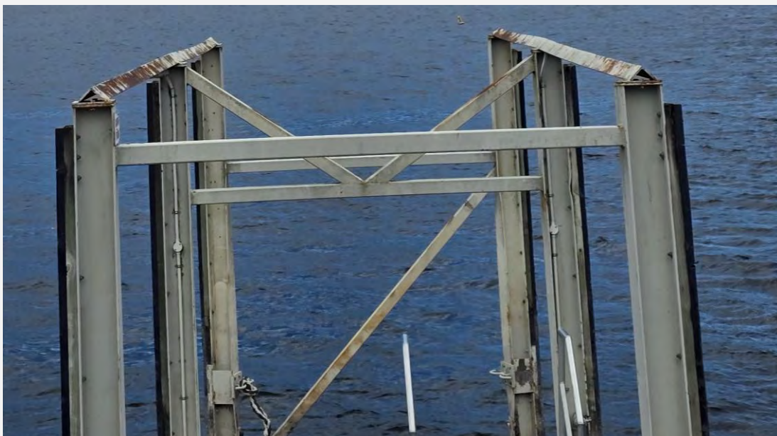
Figure 3 – photo of Real Journeys Lakefront Jetty showing bracing of the piles at the lakeward end
