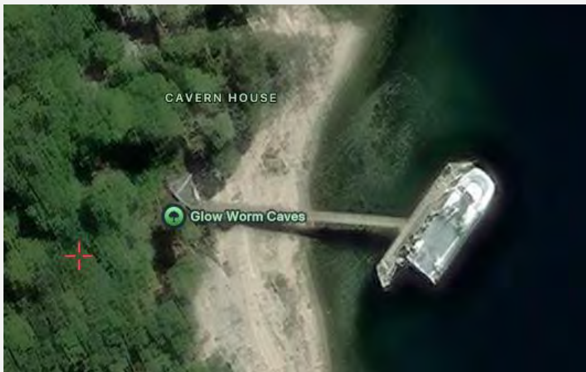
Figure 38 – aerial view showing the Luminosa alongside the Te Ana-au Glowworm Caves wharf 2
