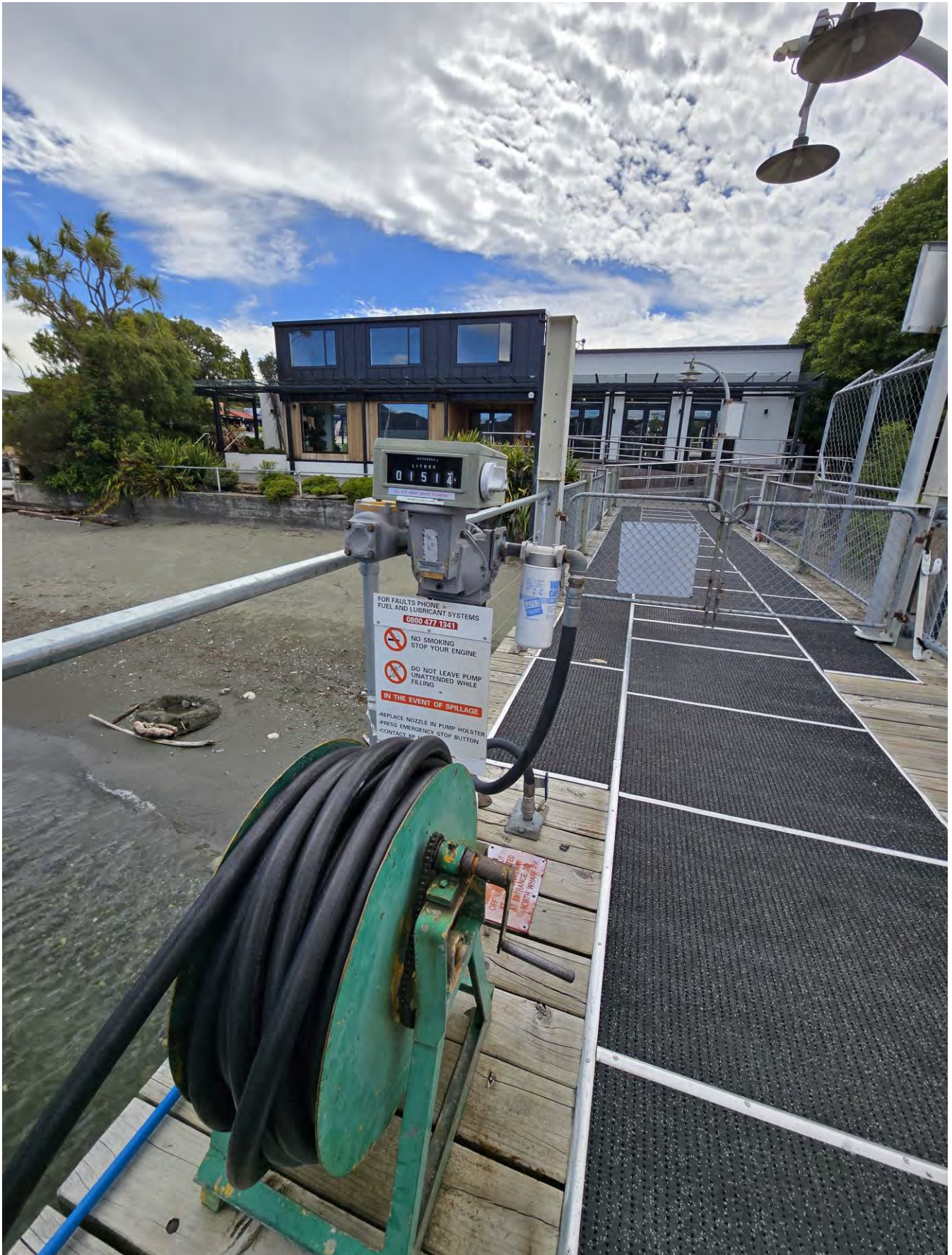
Figure 43 – photo of the landward end of the Te Anau Lakefront Jetty
