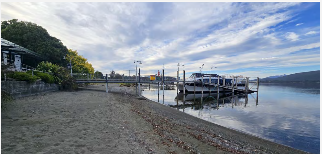
Figure 10 – Photo of Te Anau Lakefront Jetty
