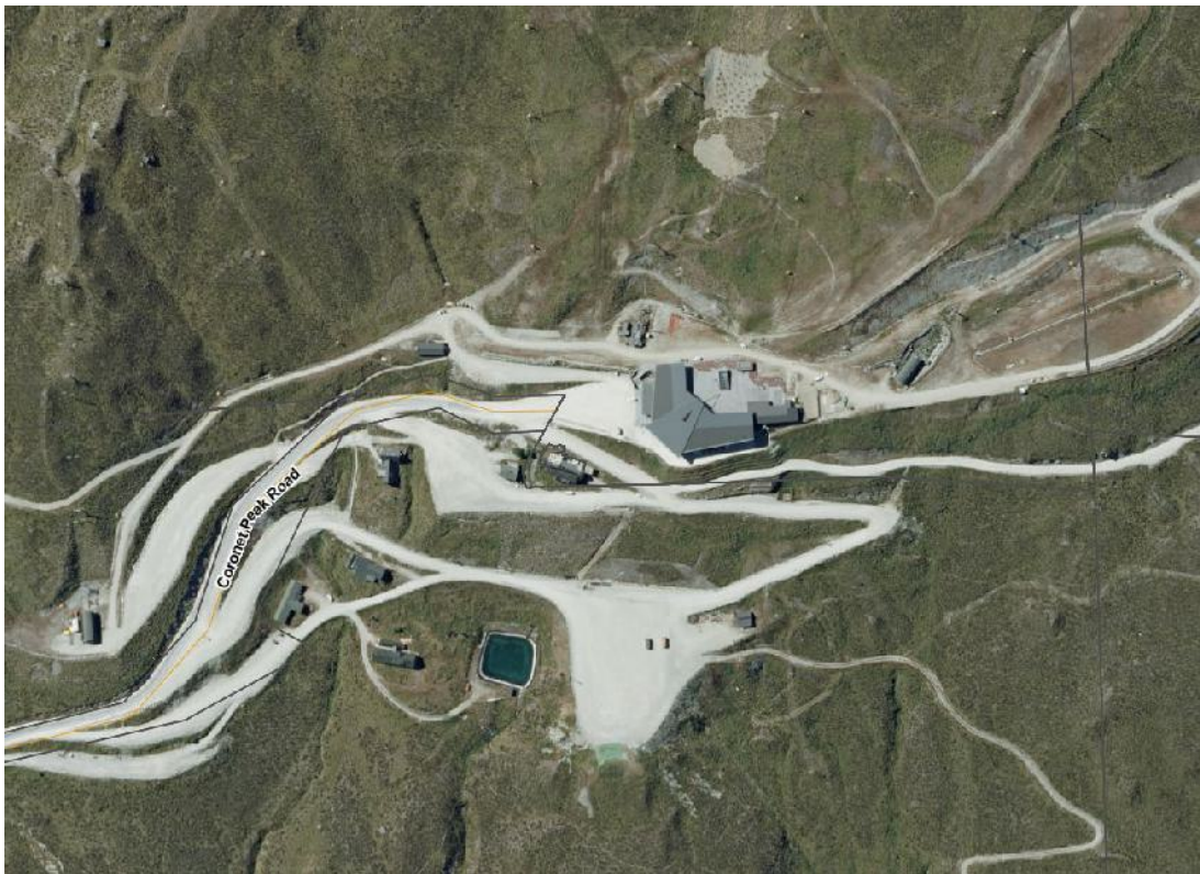
Figures 1&2: Aerials showing the Location of the Rocky Gully Hut within the Ski Field Environment (source QLDC and Google Earth).
