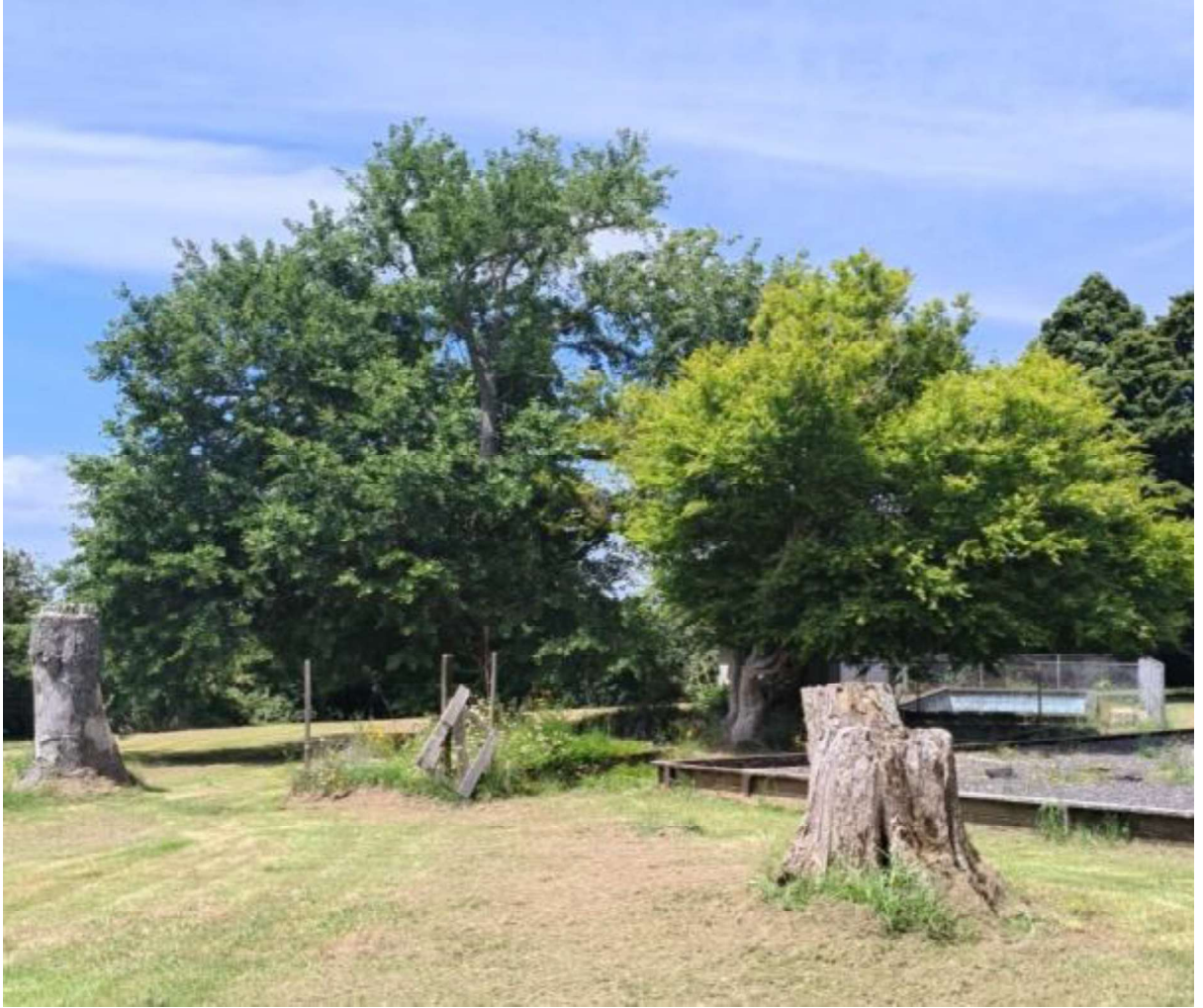
Figure 2-2d: View from existing "admin / classroom" building across "playground" area to derelict swimming pool, with northern field area to left
