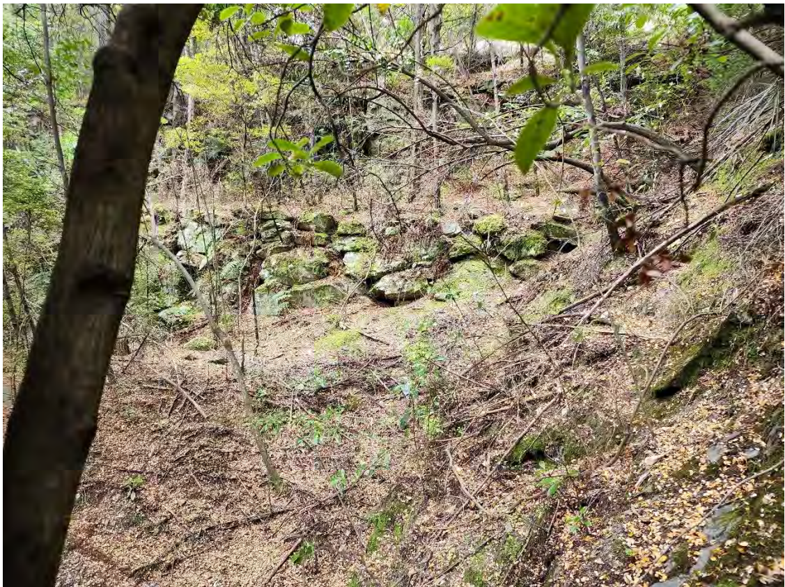
Photo 16: Benched rock wall track (WP333) west of the un-named creek which drains into the ground emerging below the benched track and rock retaining.
