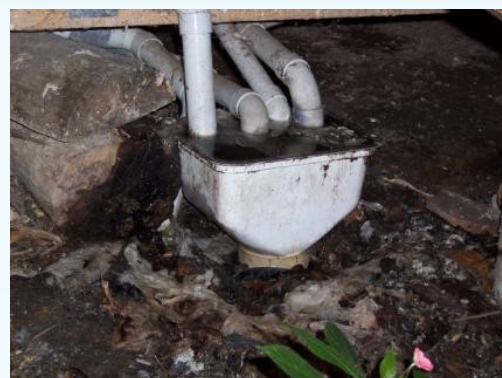
Backup to gully trap from clogged tank
