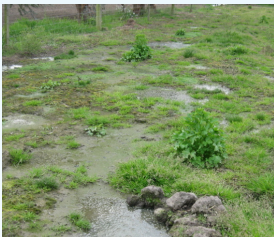
Failed soakage field
