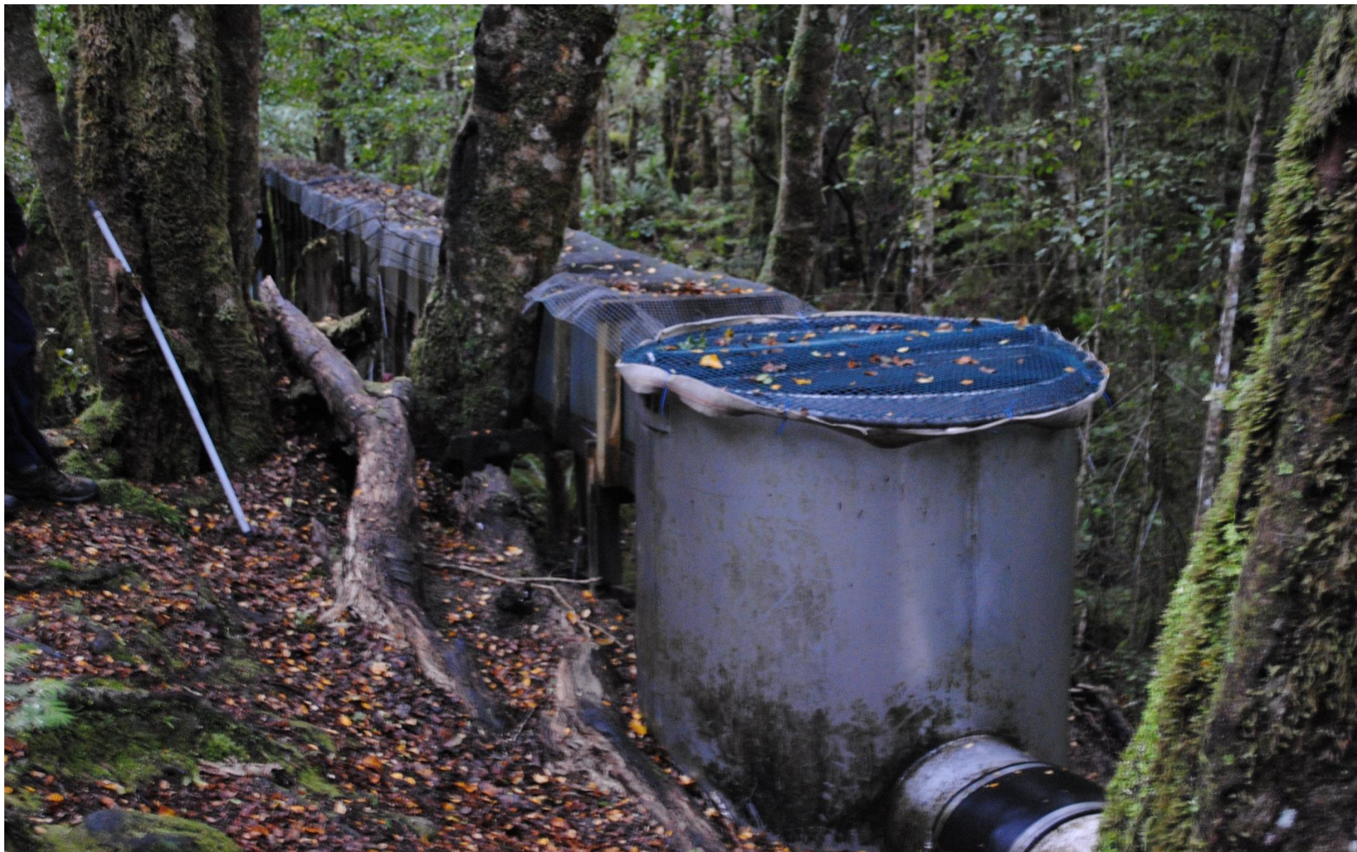
Figure 33. Photo of surge tank and the start of the hydro pipeline
