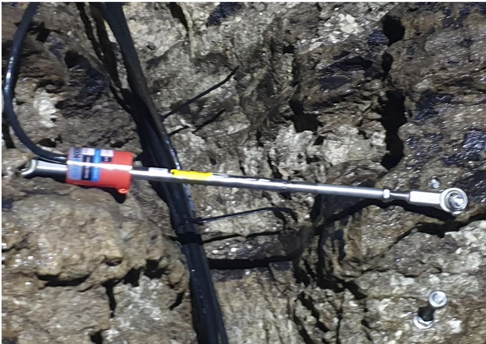
Figure 68. Further rock movement detection equipment
