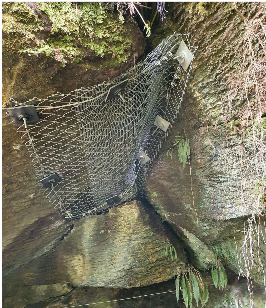
Figure 72. Cave entrance protection structures
