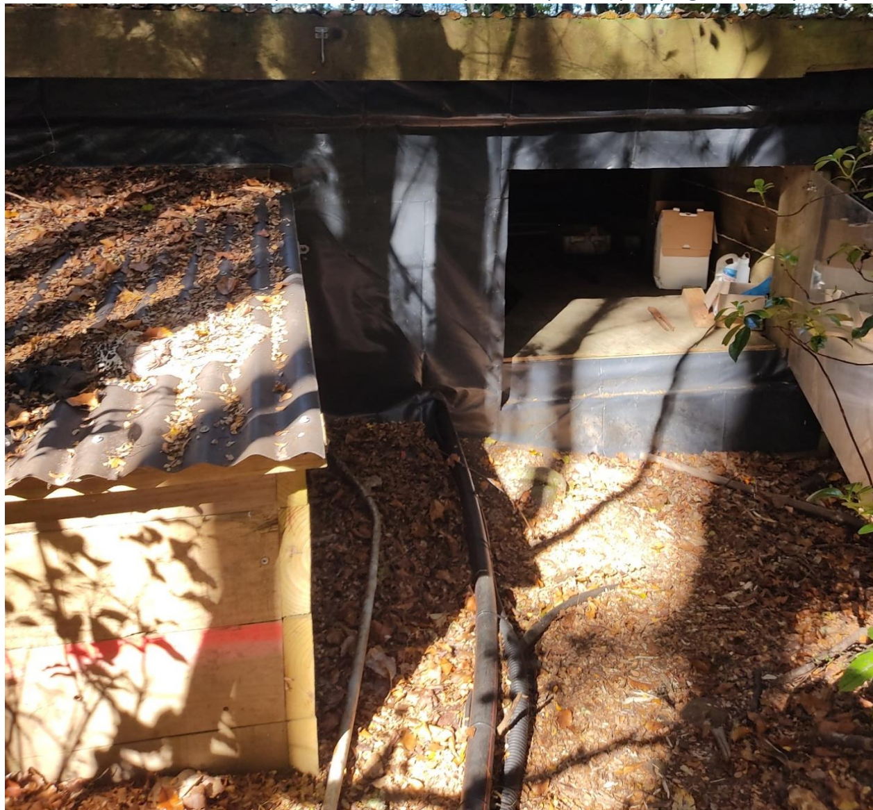
Figure 29. Photo of exterior of wastewater treatment plant pumphouse bunker (the tanks used to collect the liquid overflow from septic tank prior to pumping to AES disposal field)
