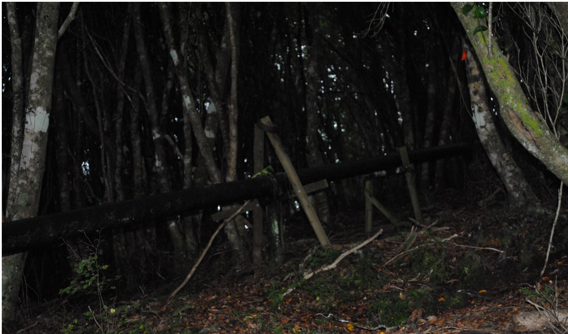
Figure 35. Photo of pipeline including support structures
