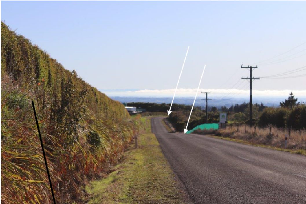
FIGURE 11 - VIEW OF EGMONT RD LOOKING NORTH EAST
