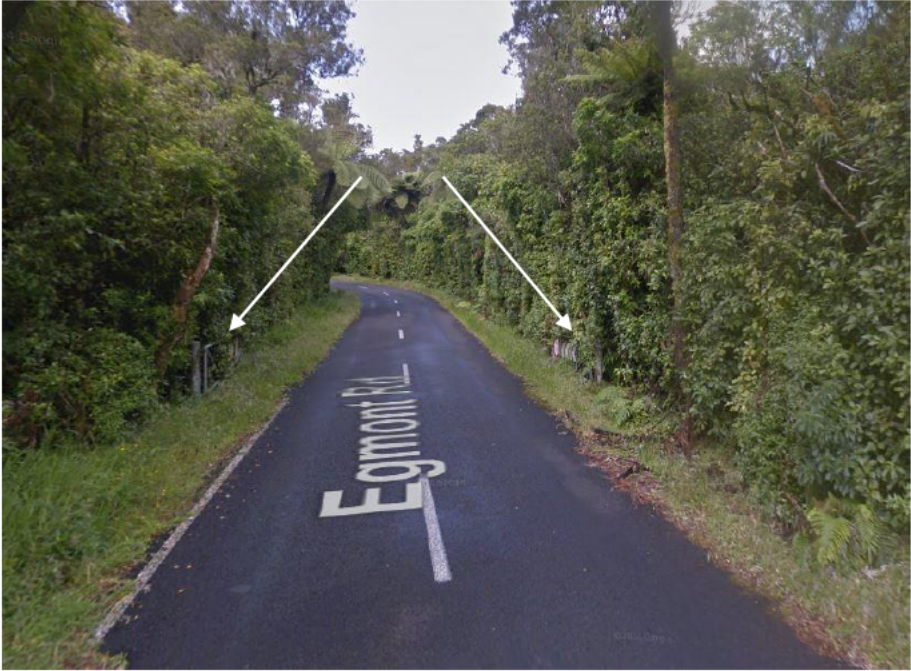
FIGURE 3 - IMAGE OF THE ROAD GATES
