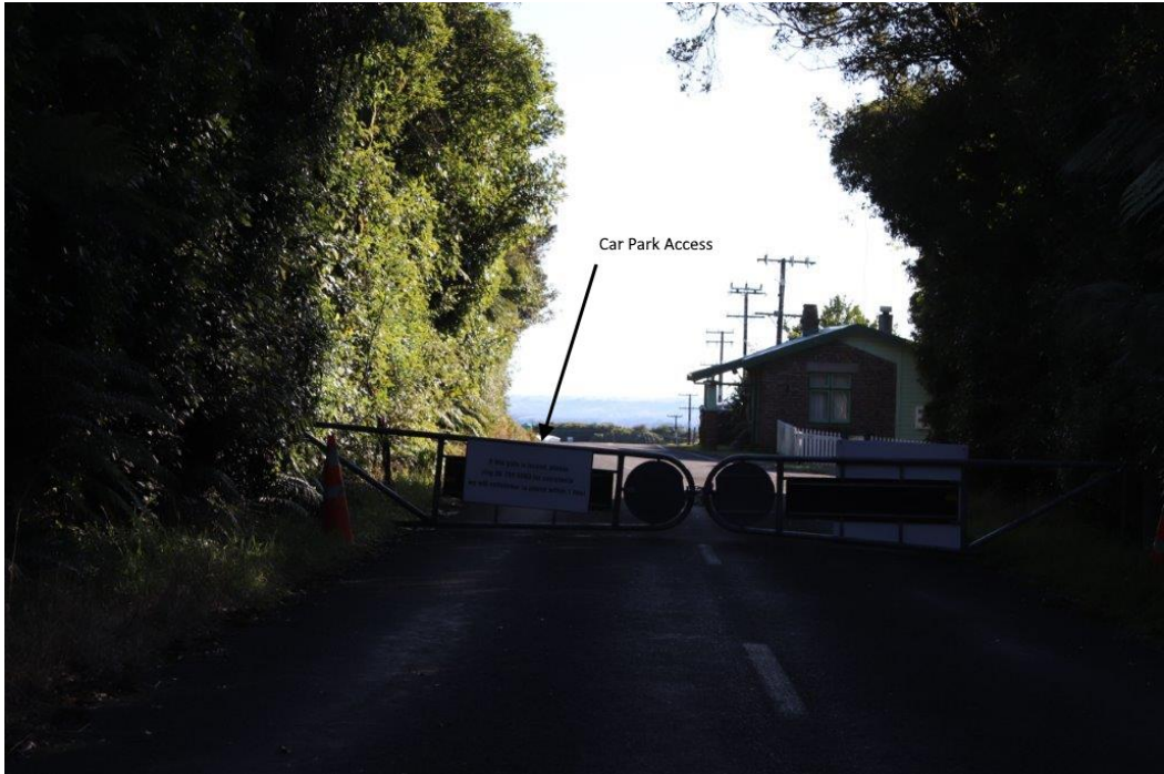
FIGURE 13 - VIEW FROM NATIONAL PARK TO CAR PARK
