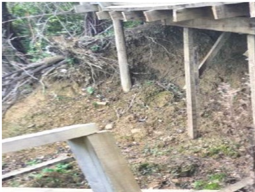
Figure 6. View of head scarp showing predominantly silt material with minor schist cobbles. Source: EDC site visit photos
