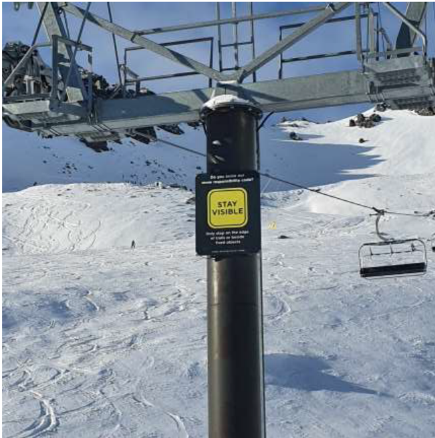
Fig 1: Example of paint colour and galvanised 'head' structure.
