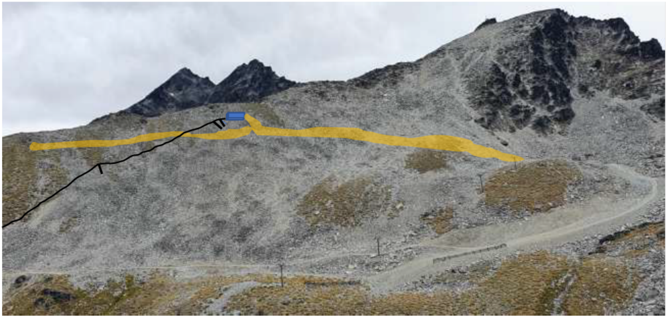
Photo above portrays top station location, Towers 8,9 & 10, Calypso & Cushion trails
