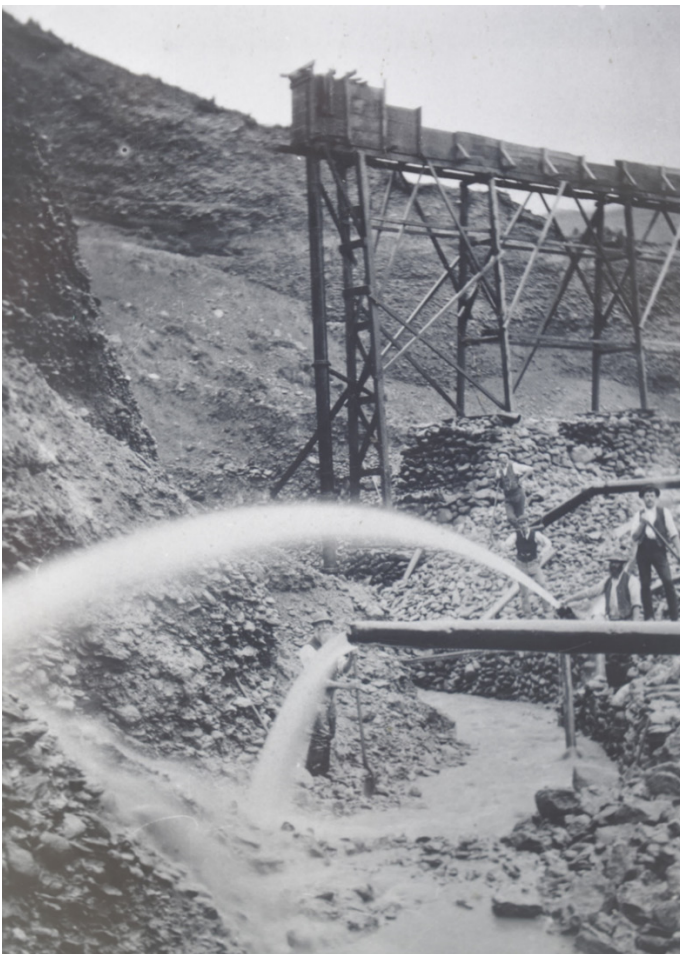
Figure 19. Hydraulic elevator sluicing at Dave Adie's claim in Lower Nevis in 1934. Photo: Louise Joyce.
