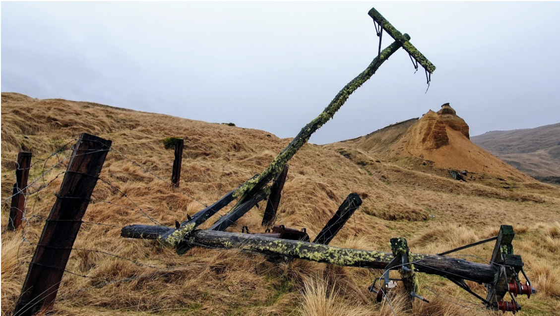
Figure 11. Old hydro-electric lines and gold sluicings, Te Papapuni/Nevis River. At Baileys Hill in the Upper Nevis, a network of three family groups worked the complex alluvial faces improvising simple electric power systems using the 19th century water races up until the late 1980s. Photo: Carl Walrond, DOC.
