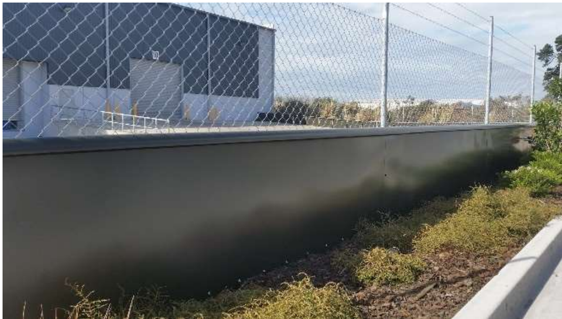
Figure 3. 'Low' or 'rodent' fences built to protect food-processing sites in the North Island.
