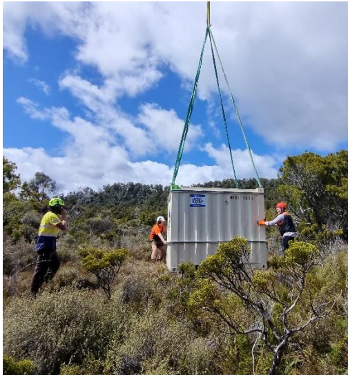
Left: Container being helicoptered into position. Right: container with floatation pontoon, solar panels and air sampling tube. Photos by John Wilks.
