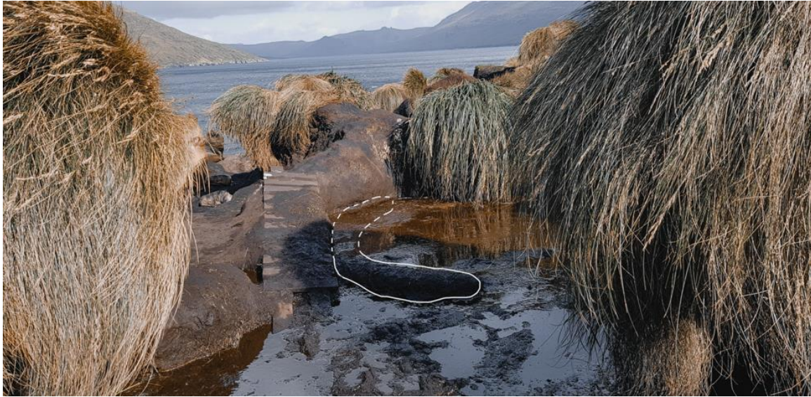
Figure 10. Giant bog showing the condition of the existing ramp installed by previous teams and the new addition of the coir log (white outline; half of it underwater as indicated by the dashed lines)
