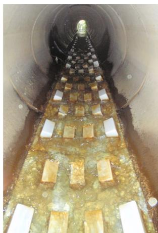
**Figure 1.** Spoiler baffle sheets installed inside a circular culvert.
