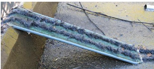
Figure 4. An aluminium ramp with astroturf lining and two mussel spat ropes installed to assist fish passage from the very beginning of the long climb ahead.
