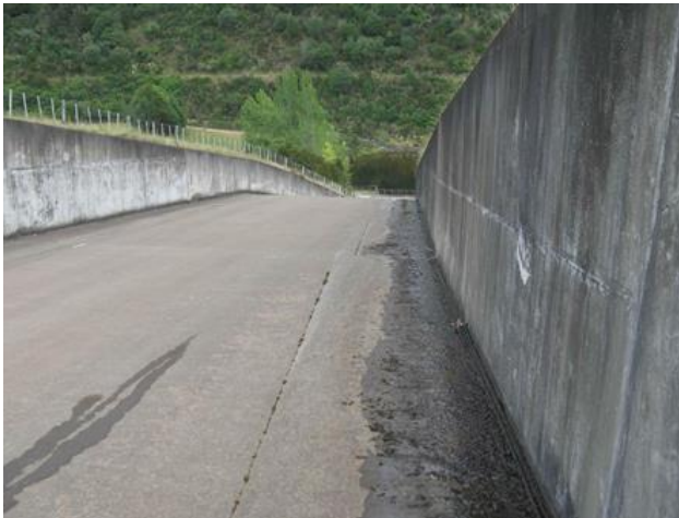
Figure 2. We installed the pump at the shady side of the spillway to ensure permanent water flow down the spillway and apron.
