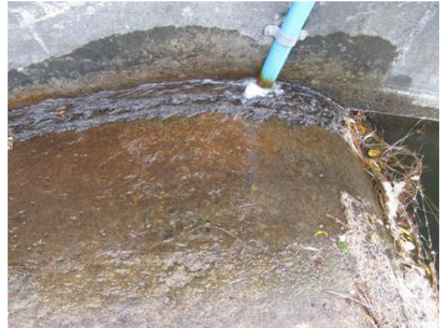
Figure 3. Mussel spat ropes installed at the shady side of the dam where the pump provides water to facilitate upstream passage of juvenile eels and kōaro.
