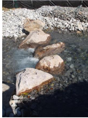
Figure 3. Side view of the upstream facing 'V' weir downstream of the culvert. (Photo: John Meikle)
