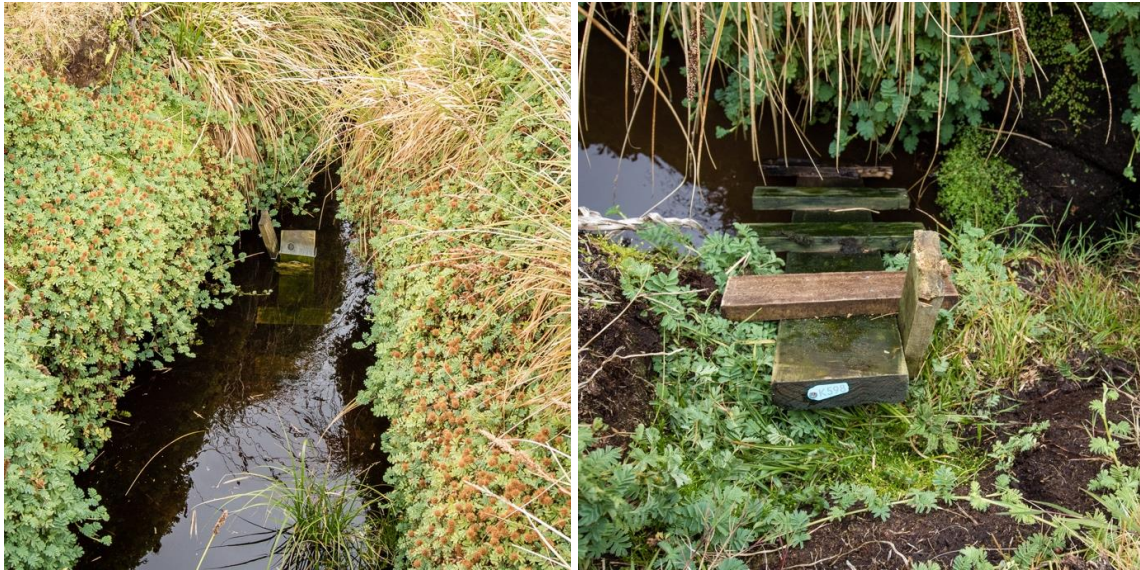
Figure A9.6 Ramp K598 at Sandy Bay, Enderby Island before alteration (left panel) and following alteration (right panel)
