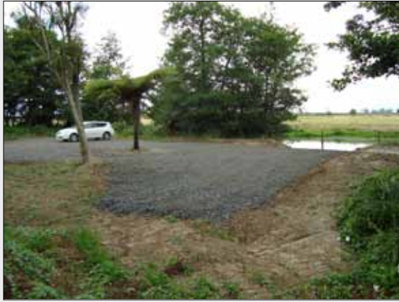
The new boat ramp at Te Onetea Stream
