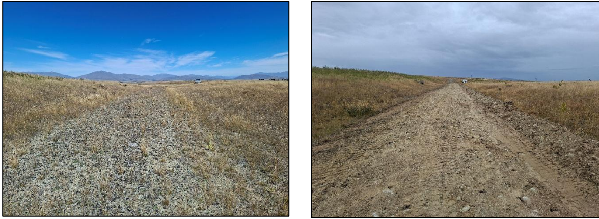
Figure 5. The Patersons Terrace road before (left) and after (right) mechanical removal of vegetation using a grader.
