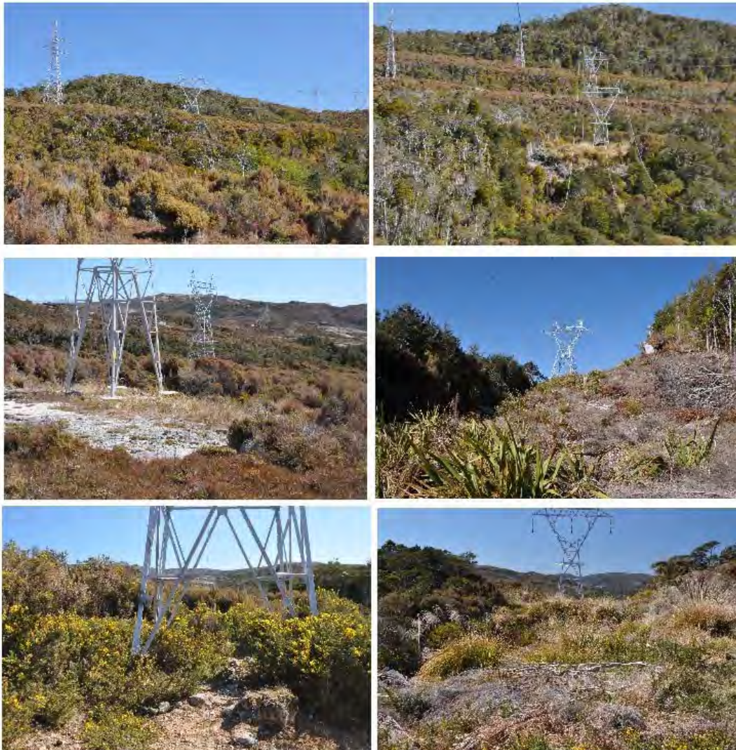
Figure 19 The impact of power lines on Powelliphanta patrickensis habitat on Denniston Plateau in 2011, where vegetation trimming under the lines has allowed sunlight to reach the litter layer and dry it out, and soil has been eroded from under the poles once the hard sandstone capping layer has been broken. Note arrival of weedy gorse. Top photos illustrate the visual intrusion transmission lines can cause in the open landscape of the Plateau, reducing the likelihood of protection of the snail habitat under it. The proposed Meridian transmission
