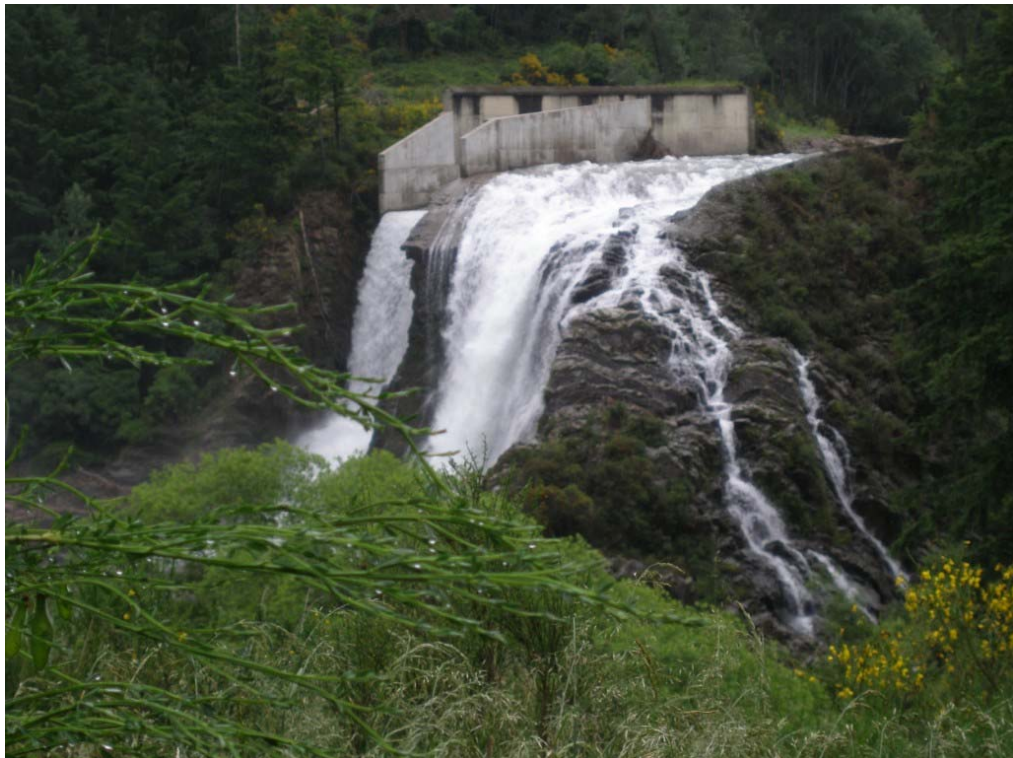
Waihopai Dam spillway with minor flood flow.
