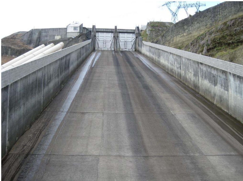
Patea Dam spillway.
